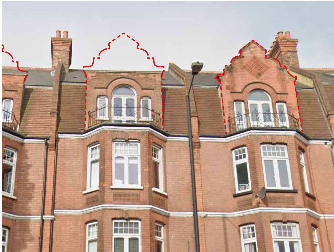
Lost decorative brick parapet above dormer of 551 -557 to be reinstated.
