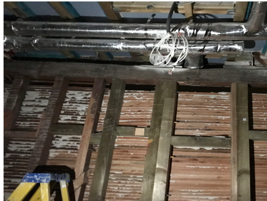
2.03 - Existing laths seen from the bathroom side, note missing laths at high level. - proposal is to use part of this gap and repair the remainder. October 2020
