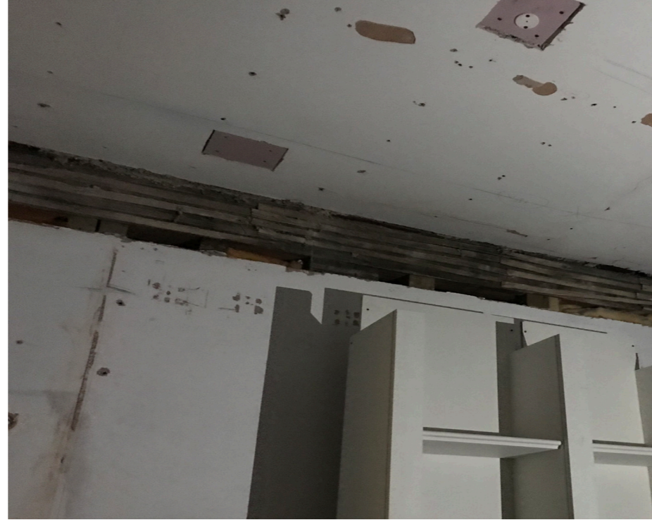
2.06 - existing lath and plaster wall with showing gaps in lath at top of plaster
