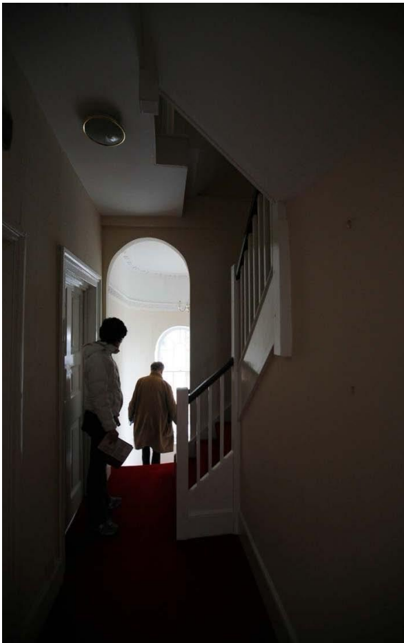
Image 31: The dark staircase enclosure of the stairs going from second to fourth floor is most unpleasant areas of the existing building. This view also shows how the existing non original stairs project into the existing second floor hall.
