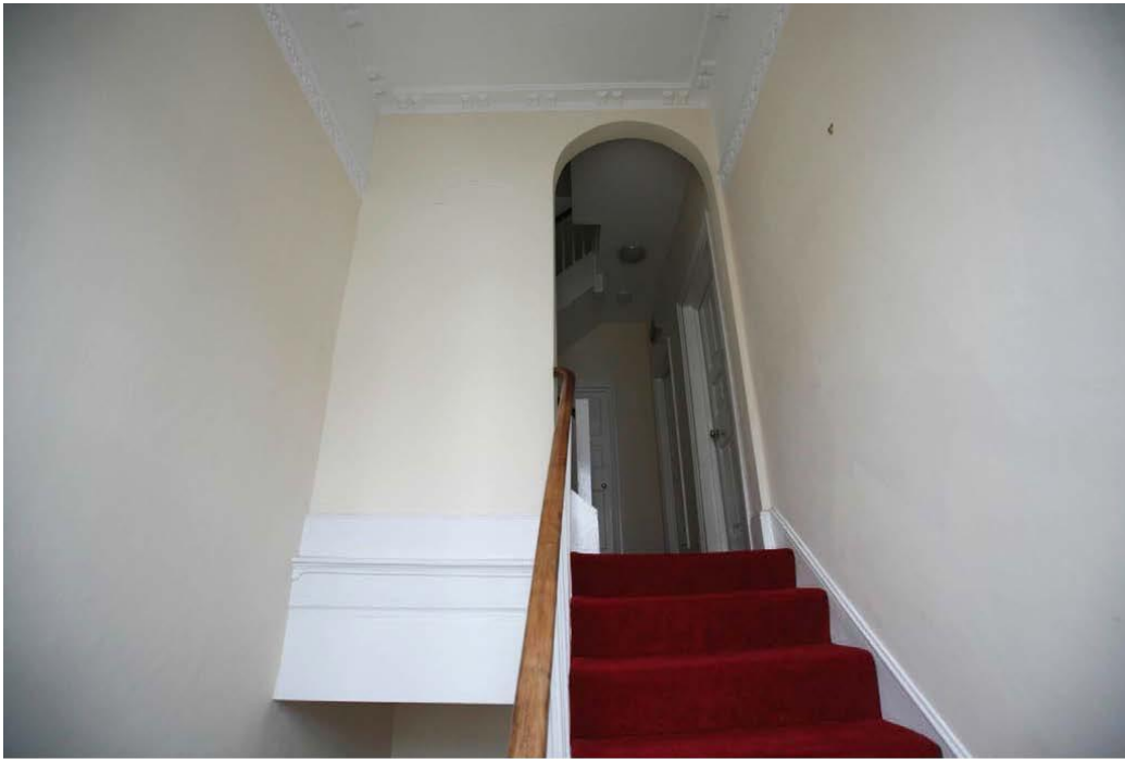
Image 30: A view to the top of the original stairs from ground to second floor showing, further in, the dark staircase enclosure of the stairs leading to the higher storeys of the house. This view also shows the junction between the original wall cornice and the non original arched partition which is proposed to be demolished in the current design proposal.
