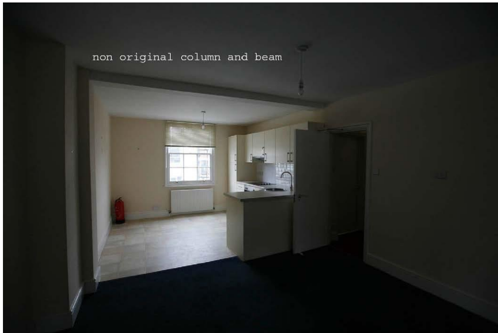
Image 32: View to non original kitchen at third floor level showing non original column and projecting beam. As is the case with the second floor, the non original structural elements at third floor level will be integrated into the design.
