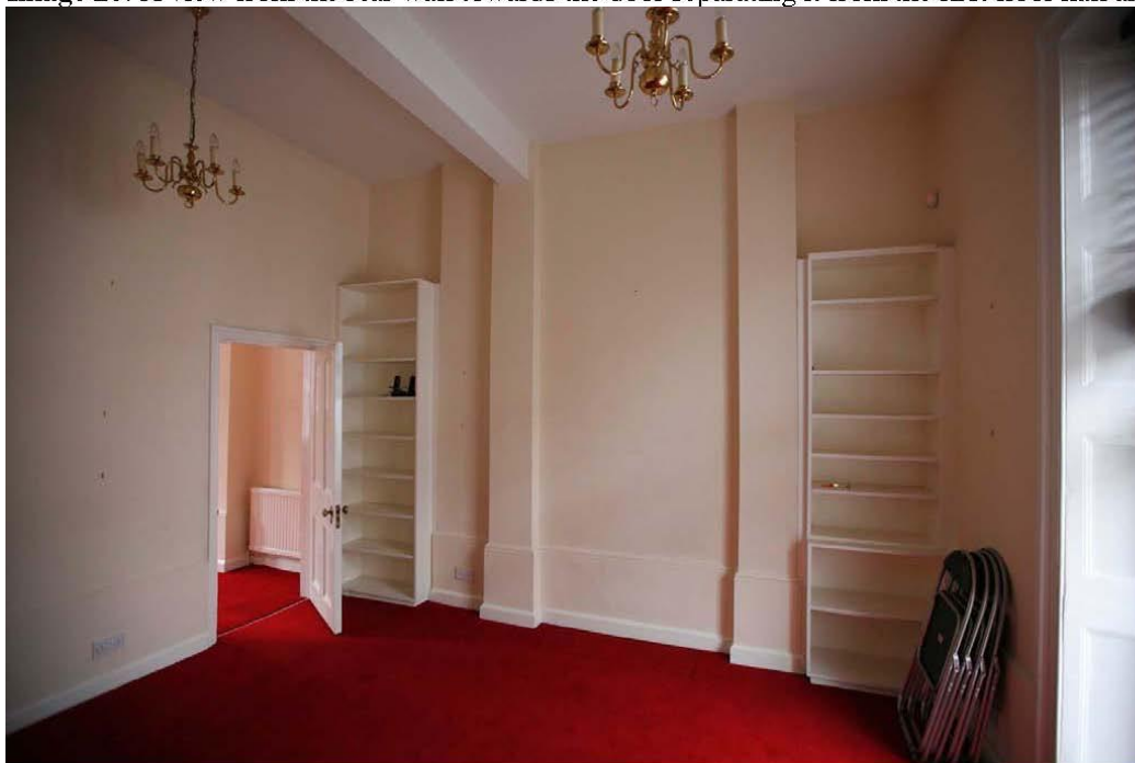
Image 25: Rear room at first floor level with non original columns in wall, projecting beam and missing fire place.
