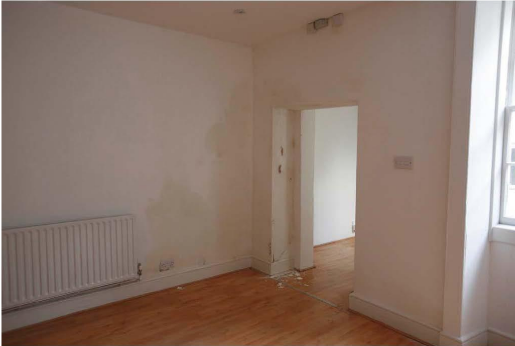
Image 13: Front basement area: non original columns; out-of-character radiators; plasterboard ceiling with spot lights; moisture on walls.
