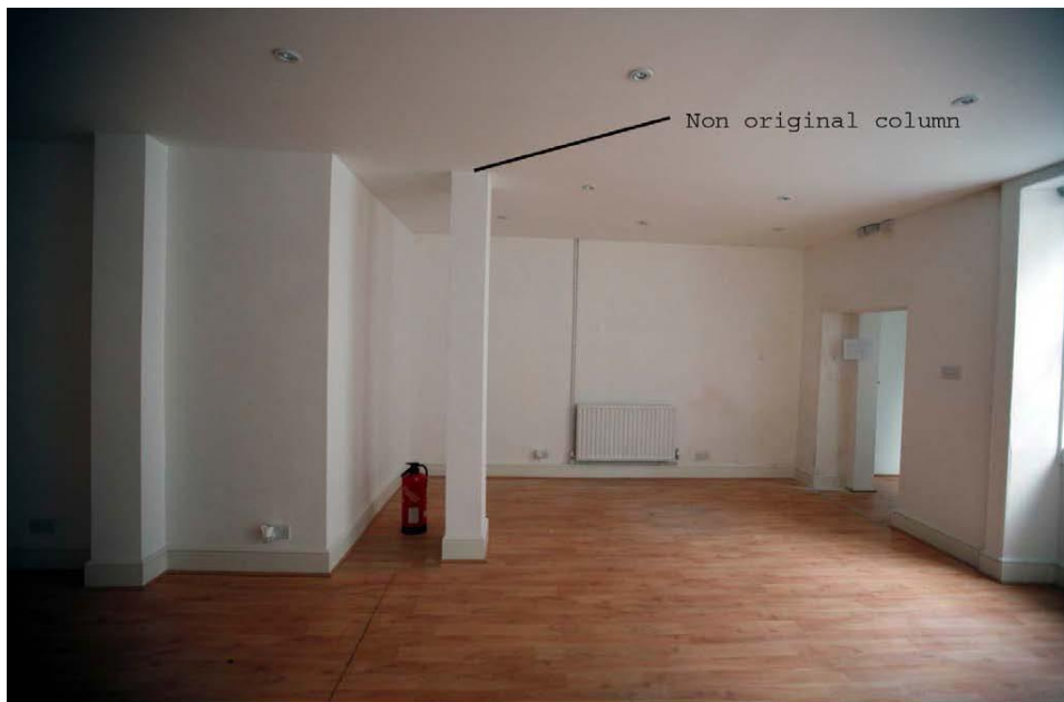
July Image 12: A non original structural column, as viewed at basement level.
