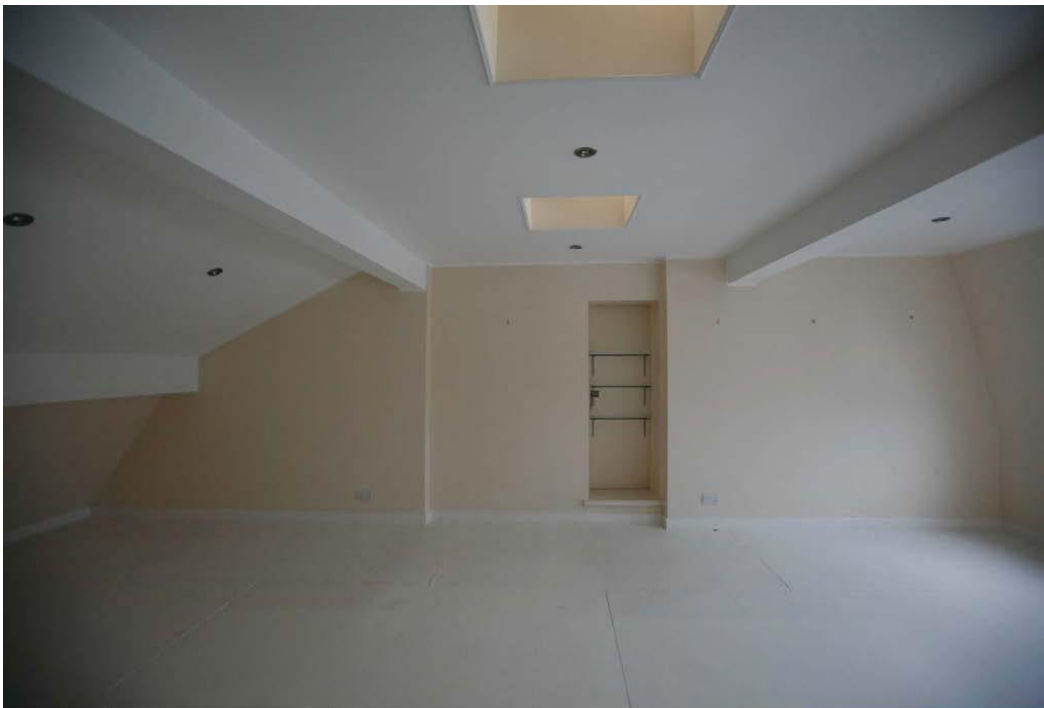
Image 37: A view to the side of the fourth floor showing the later added beams. The beams are integrated into the current design proposal.
