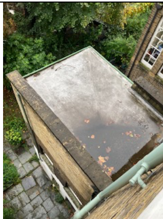
Fig 22 Replace copper roof, current design does not meet current building standards, not enough insulation and no adequate upstand.
