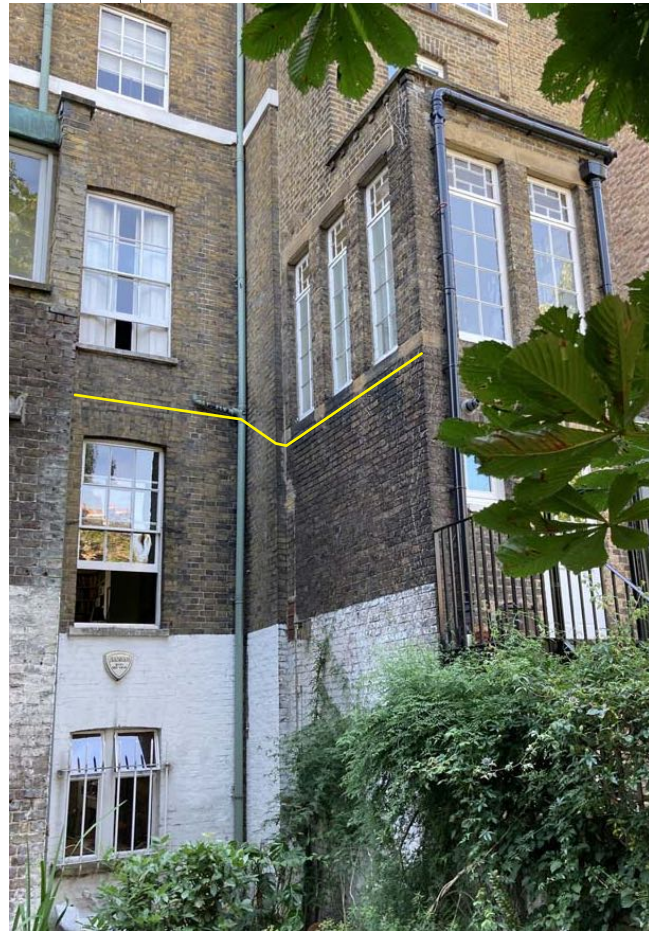
Proposed roof line highlighted in yellow. The angle fixed glazed roof light that connects the roof back to the house allows for a minimal visual harm to the existing ground floor rear window.
