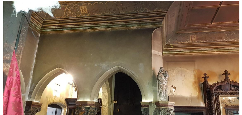
Room 2 – Additional photo of smoke damage.
