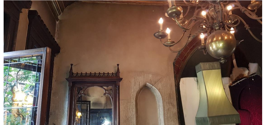
Room 2 – Wall adjacent Reception Room. Water damage and smoke staining visible
