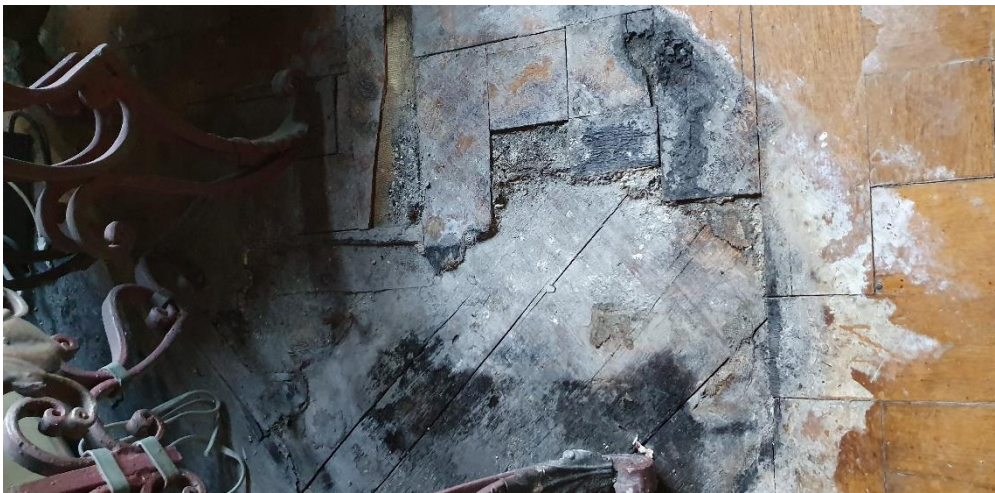
Room 1 – Damaged flooring to be removed and replaced with new
