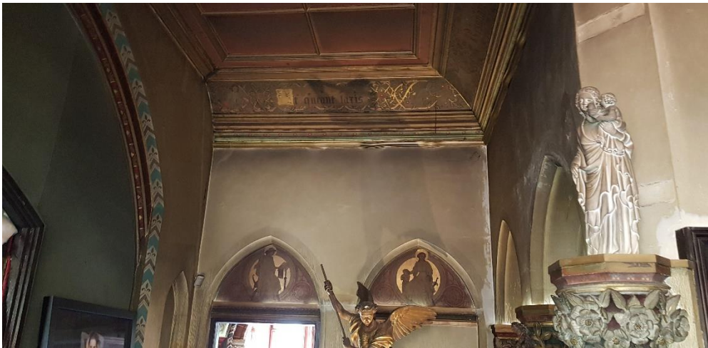
Room 2 – Example of smoke damaged decorative cornice and decorative details over door heads. Smoke damage visible to walls generally
