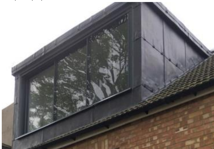
Example of proposed aluminium window frame to be used on mansard roof
