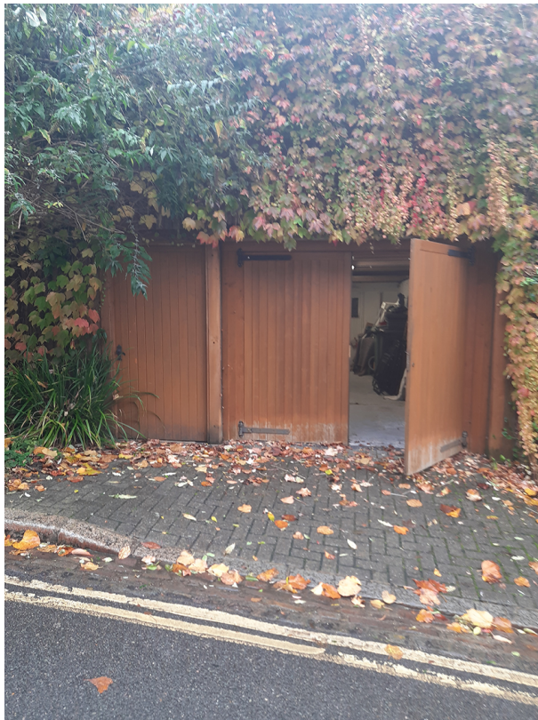
Fig 2 – Existing Garage and Garden Access
