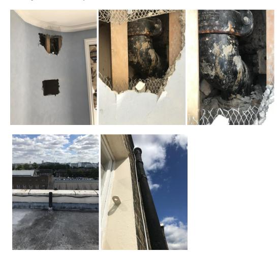
A small opening in ceiling bulkhead was made for the structural engineer to inspect the structure behind.
