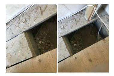
A small portion of the beams casing was removed for the structural engineer to inspect the structure behind.
