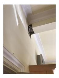
A small opening was made on both sides of the chimney breast party wall. There is a void behind enclosing SVP's and cables for the property. The wall construction is timber studs on EML mesh and plaster.
