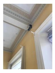
A small portion of the render above the door was removed showing a ceramic blockwork construction.
