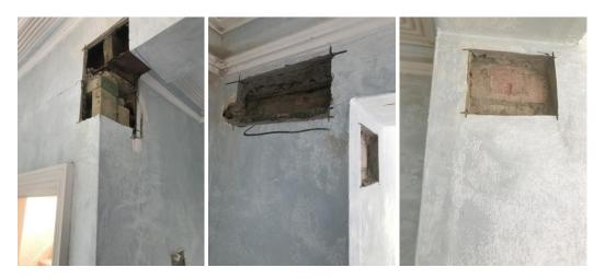
A small portion of the render was removed on the wall separating the bedroom with the hallway showing a ceramic blockwork construction.
