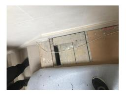
A small opening in the left hand side ceiling bulkhead was made for the structural engineer to inspect the structure behind.
