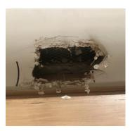
A small portion of the render in the mews wall was removed showing a brickwork construction.
