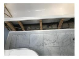
A small opening was made on the party wall to show the timber stud with EML mesh and plaster construction concealing the building service runs
