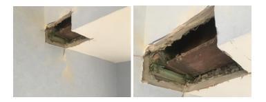
A small opening was made on the party wall to show the timber stud with EML mesh and plaster construction concealing the building service runs.
