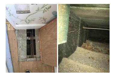
A spotlight was removed showing a non original ceiling construction
