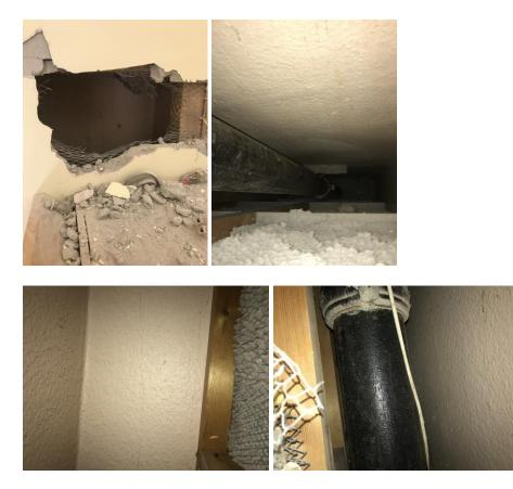
A small portion of the floor covering was removed to show a construction made of plywood on joists and revealing the ceiling on basement as a non original construction.
