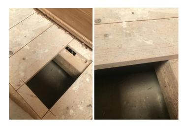
A downlight was removed to show the ceiling in this area as a non original construction.
