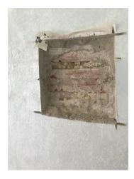
A small opening was made on the side of the chimney breast showing a newly constructed duct concealing pipes.
