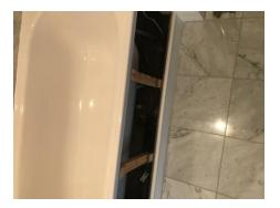
A small portion of wall coverings in party wall was removed to show the void behind with service runs and a EML mesh with plaster construction.
