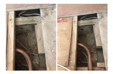
An opening both sides of the chimney breast was made showing a timber stud construction with EML mesh and plaster to concealed service runs for the building.
