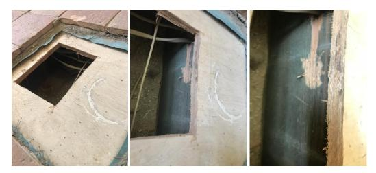
A small portion of the render on the wall between the kitchen and the water storage was removed to show the ceramic blockwork construction behind.
