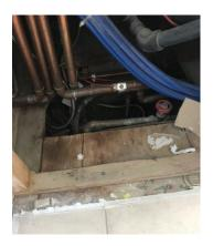
A spotlight was removed showing the non original ceiling construction.
