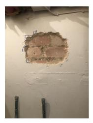
A downlight was removed to reveal that the ceiling is a non original construction.
