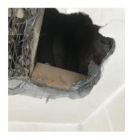
A small opening in the left hand side ceiling bulkhead was made for the structural engineer to inspect the structure behind. It showed also the ceramic blockwork construction of the internal walls on this floor.
