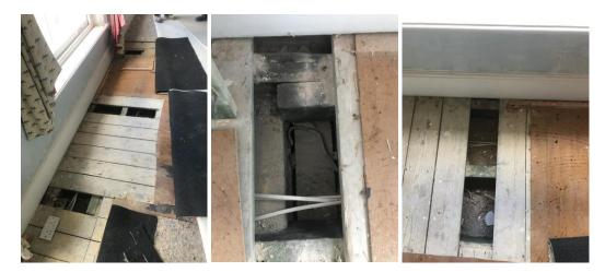
Small opening where made at the connection of the beam with the walls for the structural engineer to inspect the structure behind.
