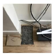
A small portion of the duct in the corner was removed. It conceals water pipes and made of timber battens with an EML mesh and render.
