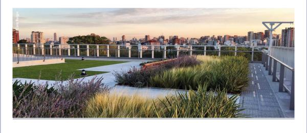
Intensive roofs traditionally require higher levels of maintenance, regular irrigation and applications of fertiliser. Due to the plants used, and the combined growing and drainage properties of the substrate, the weight of the intensive green roof system can be considerable. Substantial reinforcement of an existing roof structure or inclusion of extra building structural support may be required.
