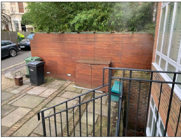
Existing North boundary photograph
