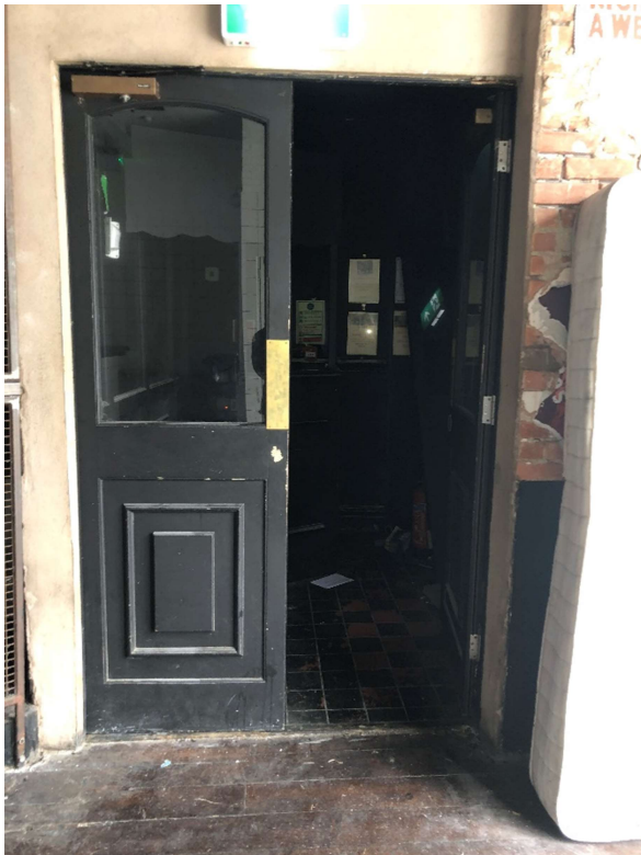
Photo 2: Existing front entrance door
