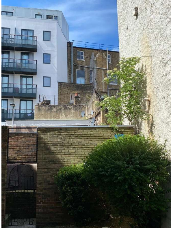
Photo 3: Existing rear access
