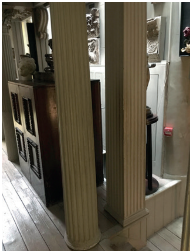
Figure 24 (Top Left): Colonnade north east columns west of Basement Stairs (top), 2019
