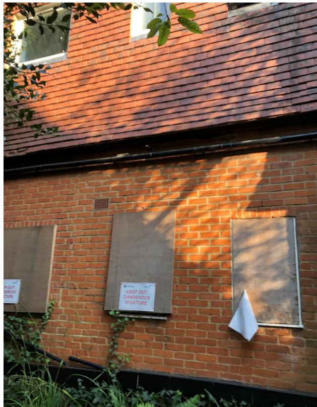
Photo 24 - South side elevation of rear extension
