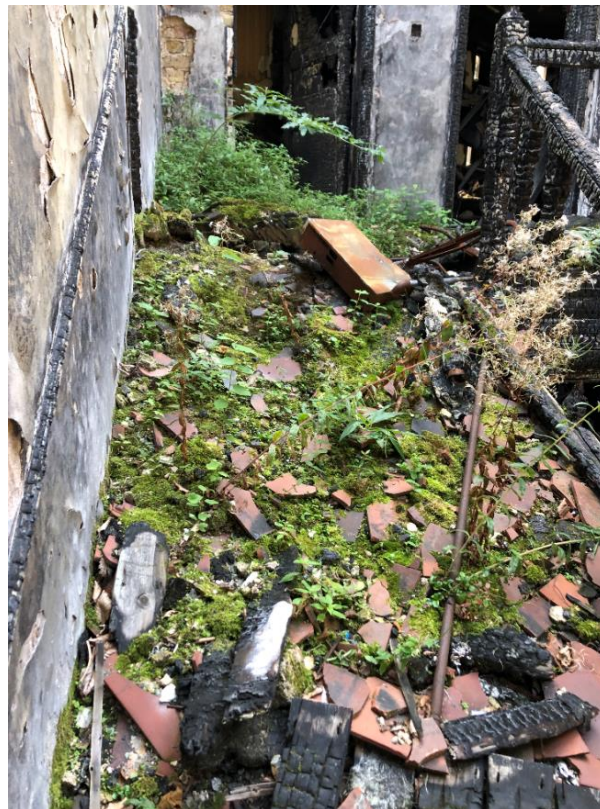
Photo 16 - Stair from ground floor to first floor
