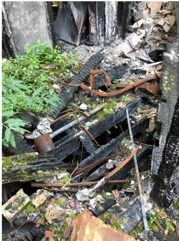
Photo 18 - First floor landing
