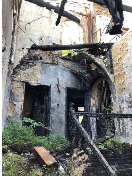
Photo 17 - Stair from ground to first floor
