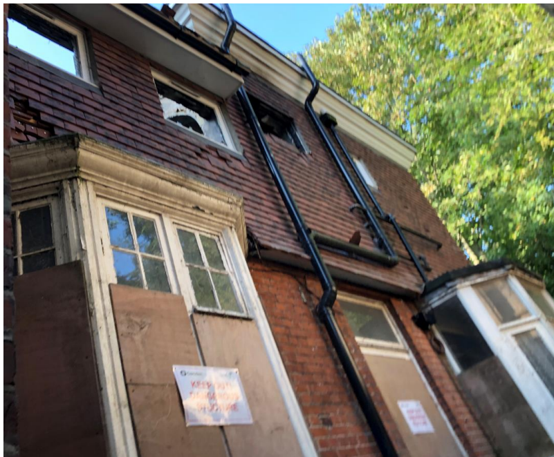
Photo 22 - North side elevation of rear extension
