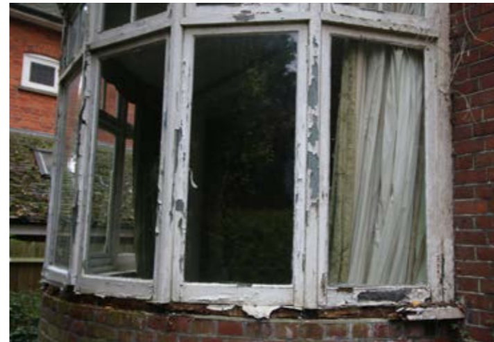
Current condition of the bay window
