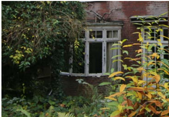
Rear View to the non-original bay window
