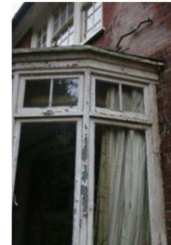
Current condition of the bay window
