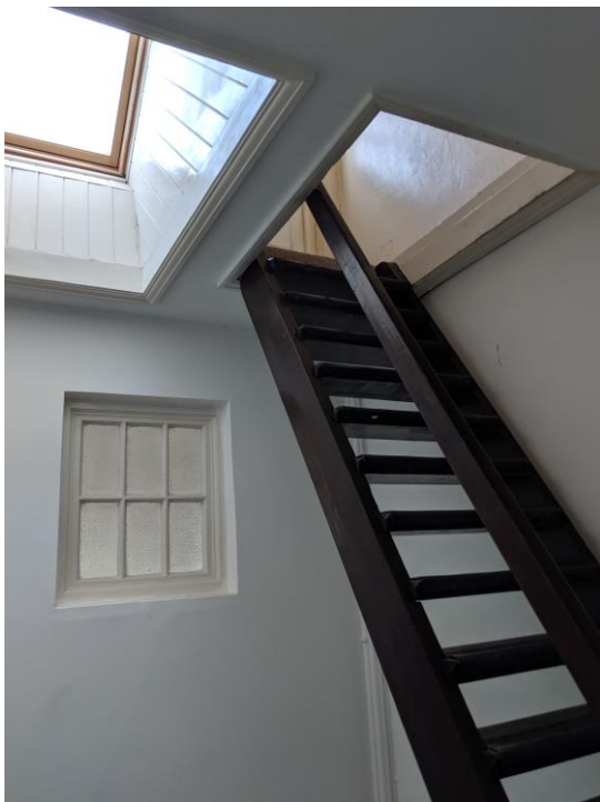
fig. 1: existing stairs and access hatch to roof terrace.
