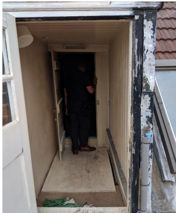
fig. 2: existing restricted doors and access to roof terrace and loft store.
