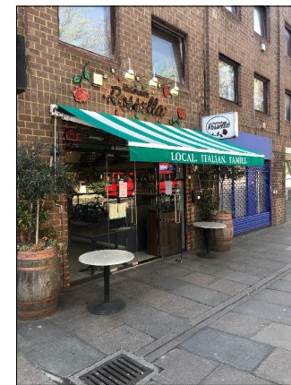
Image 1 Existing shop fronts Units 103-105 Extended awning
