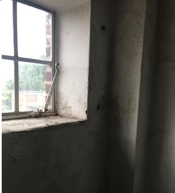
Walls to staircase A
