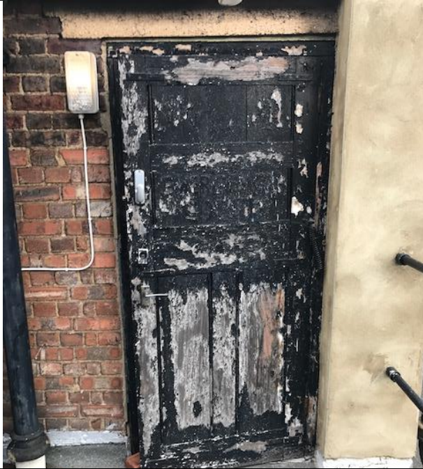
Door leading from staircase A onto roof
