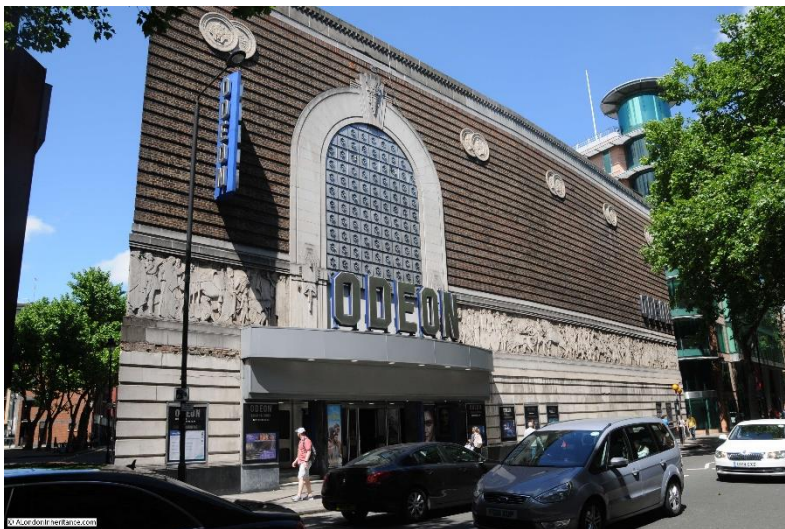
Figure 3 Front elevation of the building. Source: Flickr.
