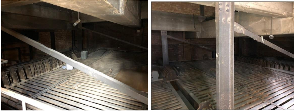
Figure 18 Photos of existing fly grid
