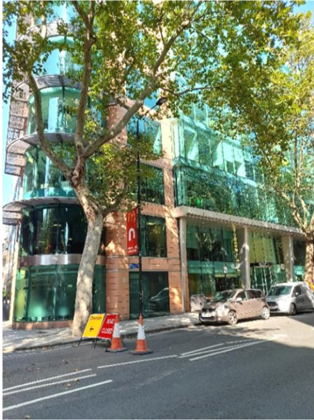
Figure 25 151 Shaftesbury Avenue demonstrating unsuccessful use of glazing.
