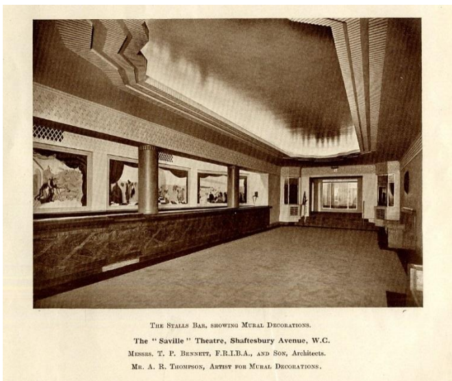
Figure 14 Stalls Bar. Source: Architects Journal.
