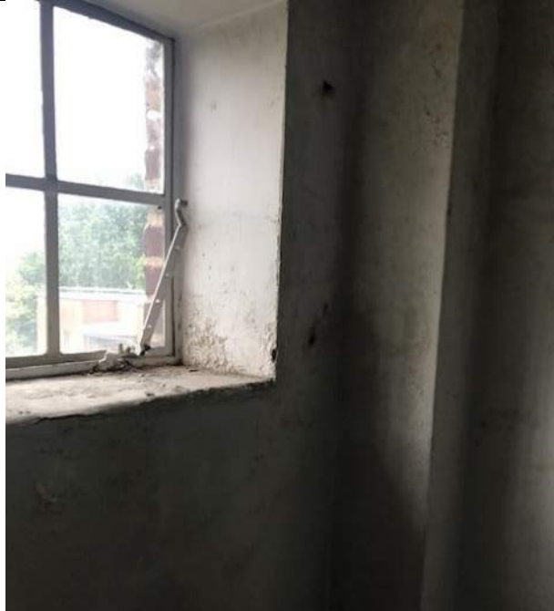
Walls to staircase A
