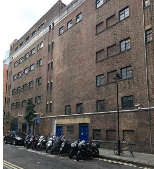
General view of rear elevation showing metal windows.
