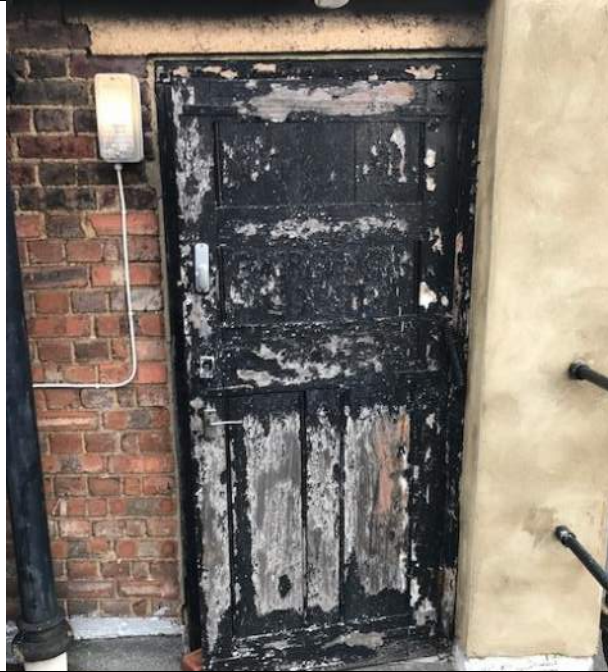
Door leading from staircase A onto roof
