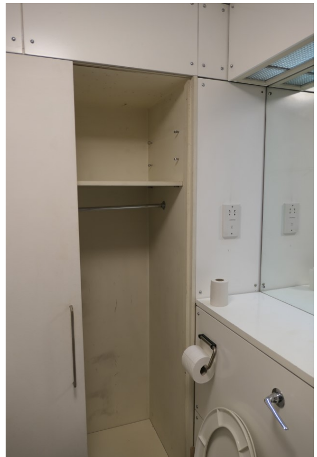
Existing bathroom at second floor
