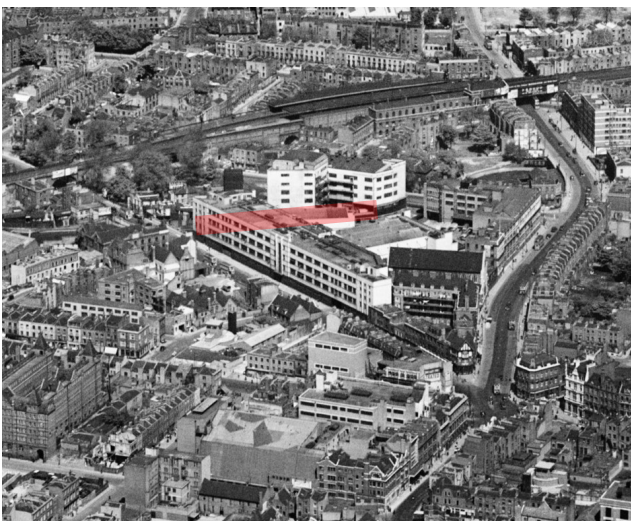
1952 aerial photograph showing the former commercial buildings of the Aerated Bread Company. The approximate footprint of 1-12 Grand Union Walk is shown as a red tone.
