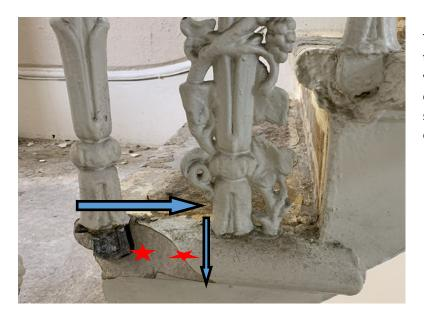
This photograph shows the typical damage to the Portland stone tread of the cantilevered staircase. The damage has been caused by the base of the iron balustrade spalling and bursting the stone at its weakess point.
