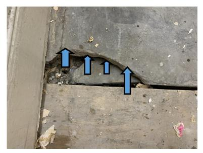
The blue arrows indicate where the new stainless steel dowels will be inserted.
