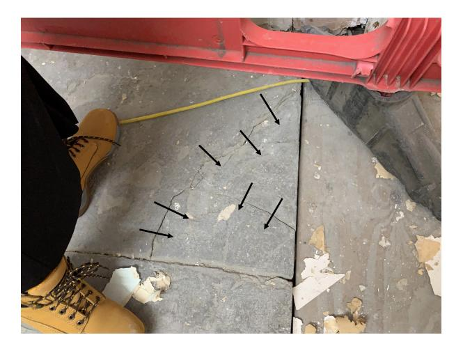
To the second floor landing the broken slab of York stone will be re-bedded as previously and have multiple pins inserted across the various cracks. The surface joints will be grouted with lime mortar.
