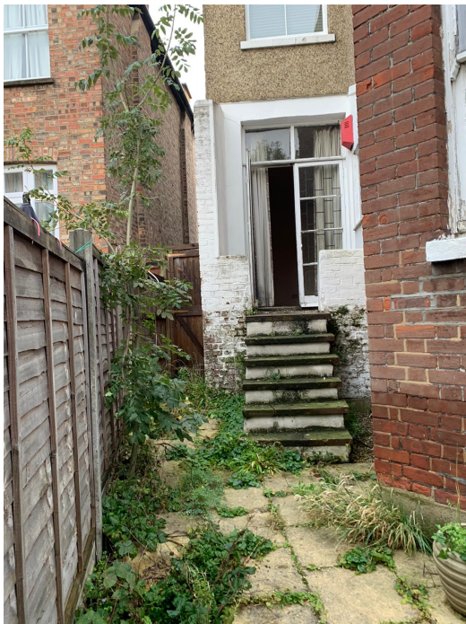
PHOTO 3 - rear side return, lane and adjoining neighbours at no. 15
