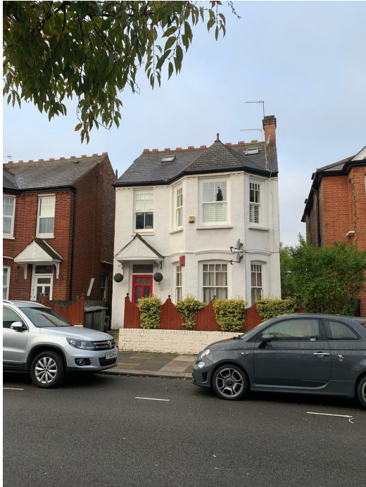
PHOTO 1 – Site - front facade
