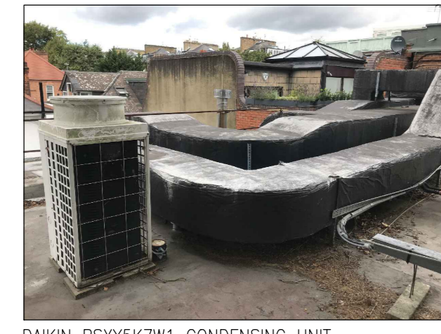
DAIKIN RSXY5K7M1 CONDENSING UNIT ANTICIPATED SOUND PRESSURE LEVEL: 54dB(A) AT 1m DISTANCE/1.5m AFFL
