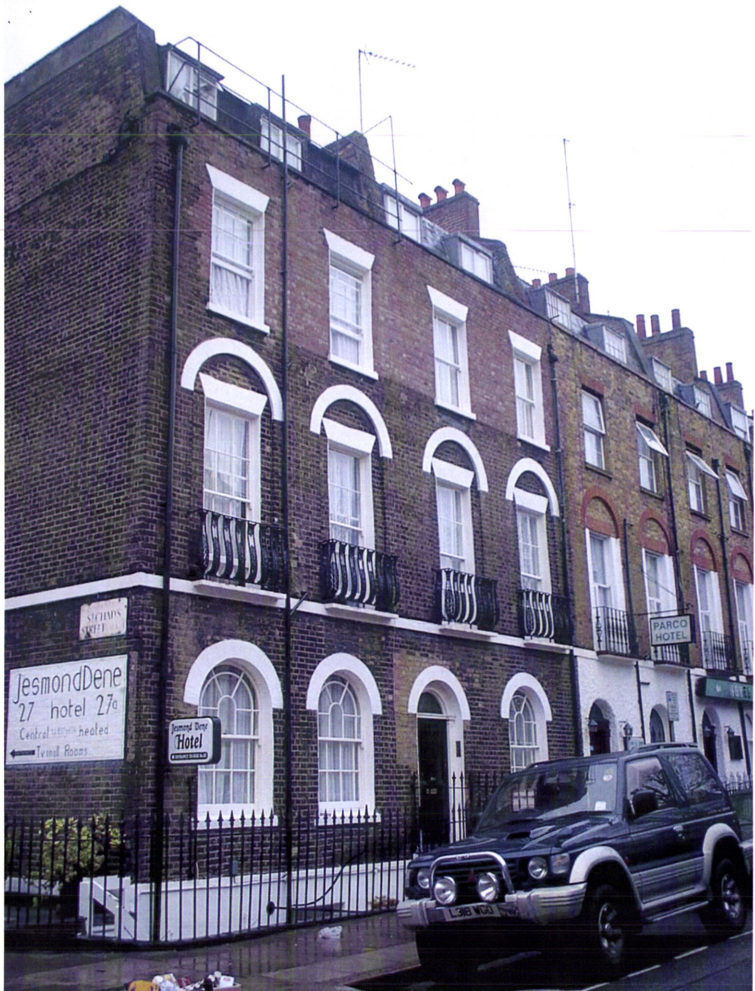
Front Elevation N o 27 Argyle Street
