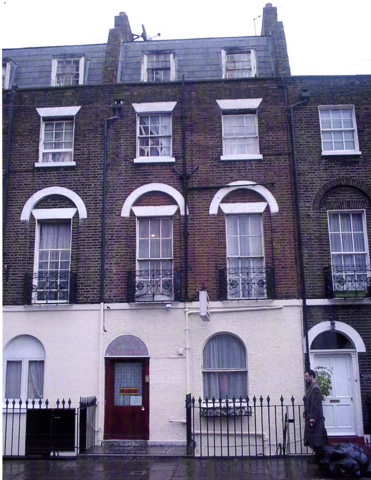
FRONT ELEVATION N o 9 ARGYLE STREET
