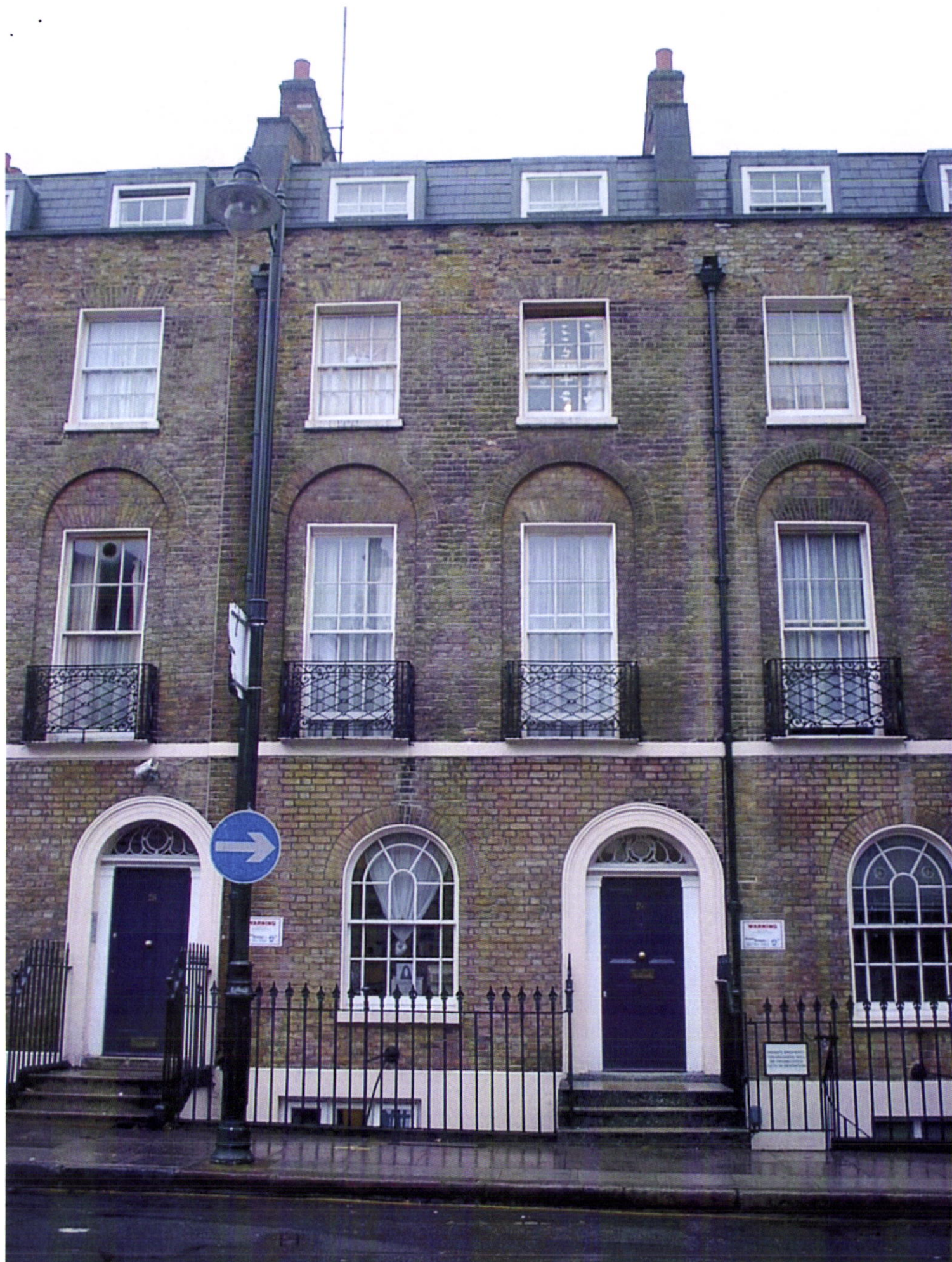
FRONT ELEVATION N o 26 ARGYLE STREET
