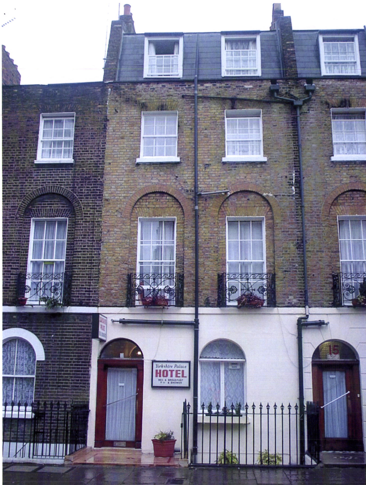
FRONT ELEVATION N o 13 ARGYLE STREET
