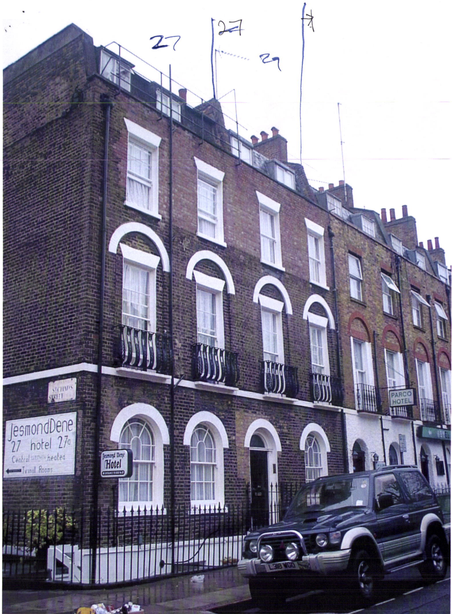
FRONT ELEVATION N o 27 28 Argyle Street + 29.
