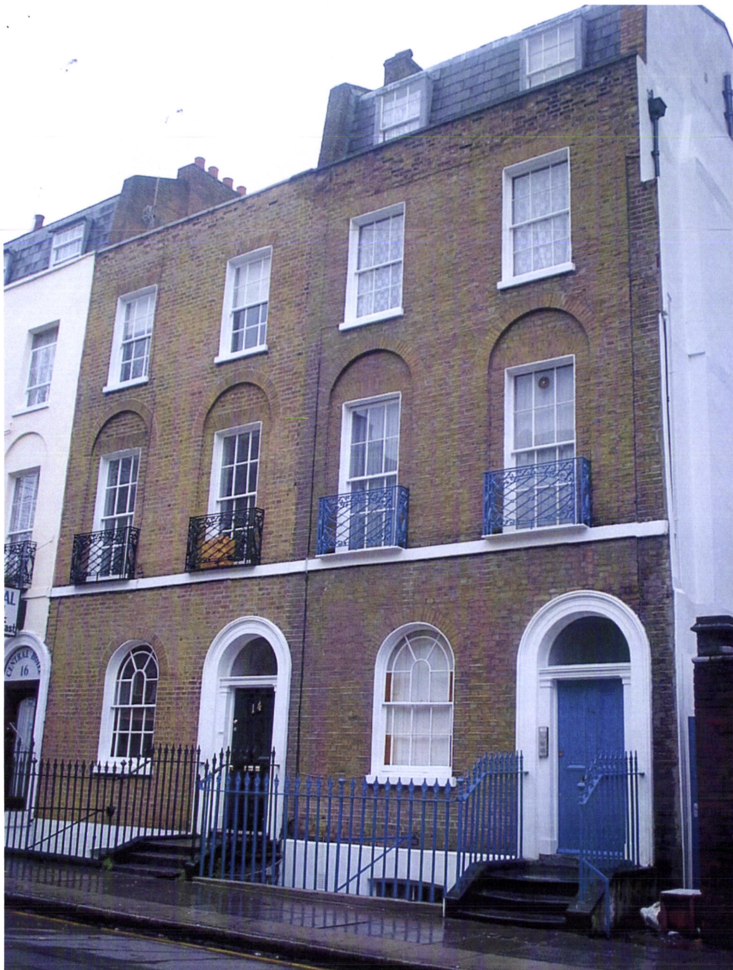
FRONT ELEVATION N o 12 ARGYLE STREET
