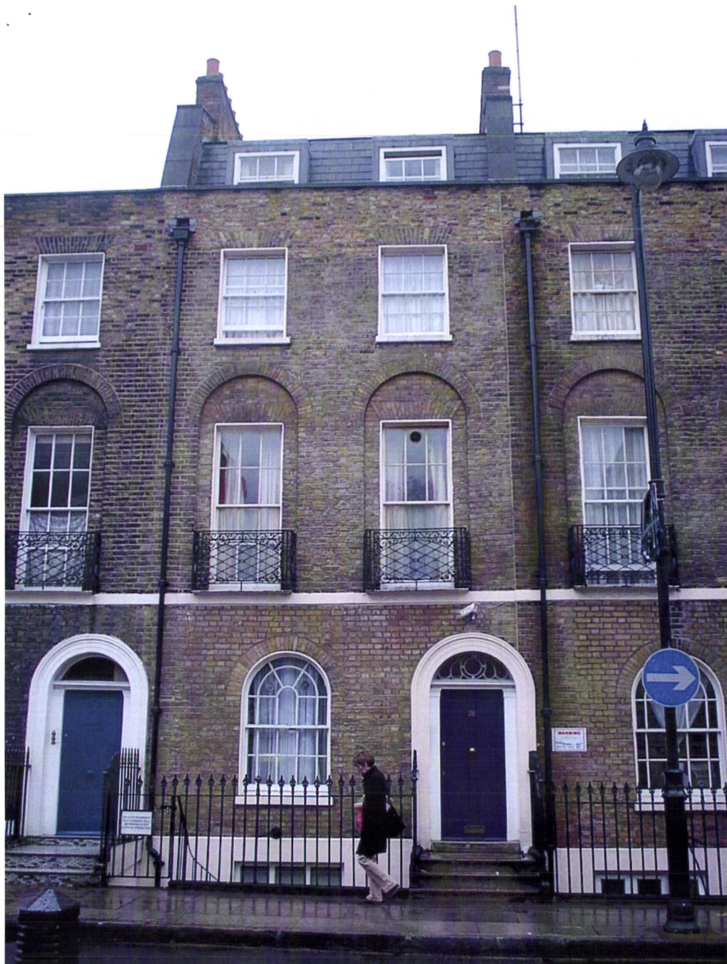
FRONT ELEVATION N o 28 ARGYLE STREET
