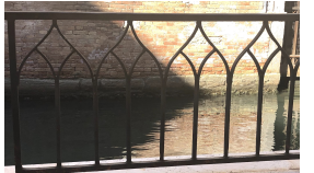
IMAGE 1: New balustrade style at first floor rear terrace. The openings will be smaller than in this image so that it complies with Building Regulations (100mm sphere must not be able to pass through any opening)
