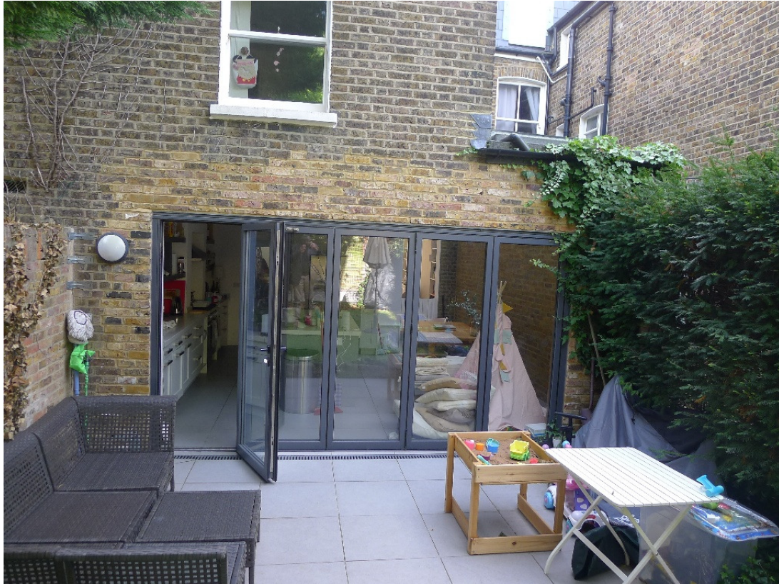
Rear view of existing side extension to number 8 Ulysses Road
