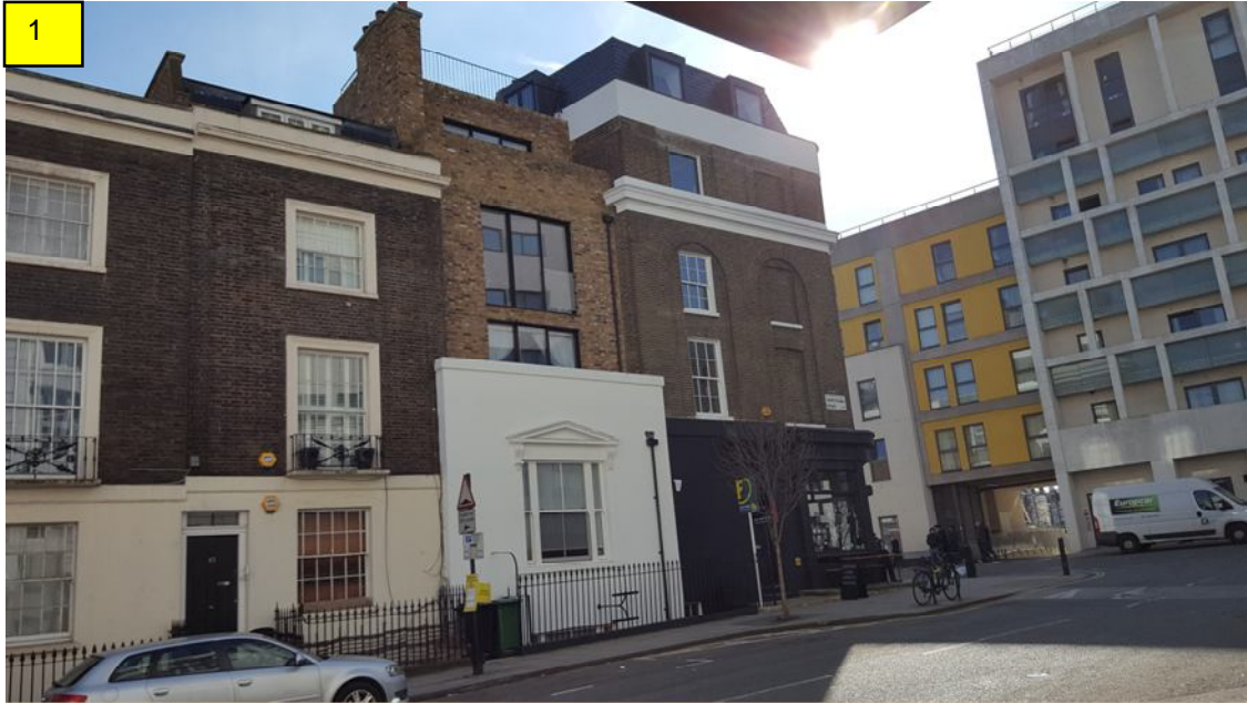
Photo 1 Photo showing the new infill extension as built adjacent to the original building with the mansard roof extension from Jamestown Road. The glazed screen proposed at roof level on top of the new infill extension will not be visible at all from Jamestown Road.
