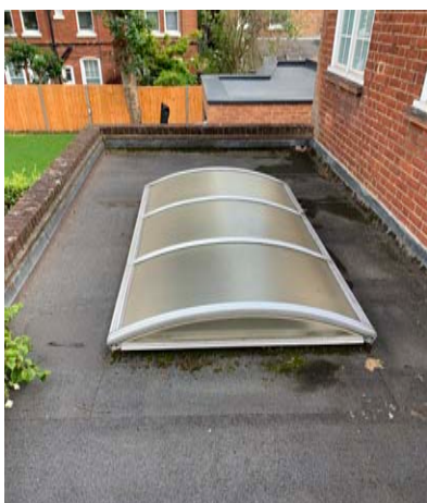
Photo of the existing rooflights over the ground floor extension (proposed to be replaced - item 3).
