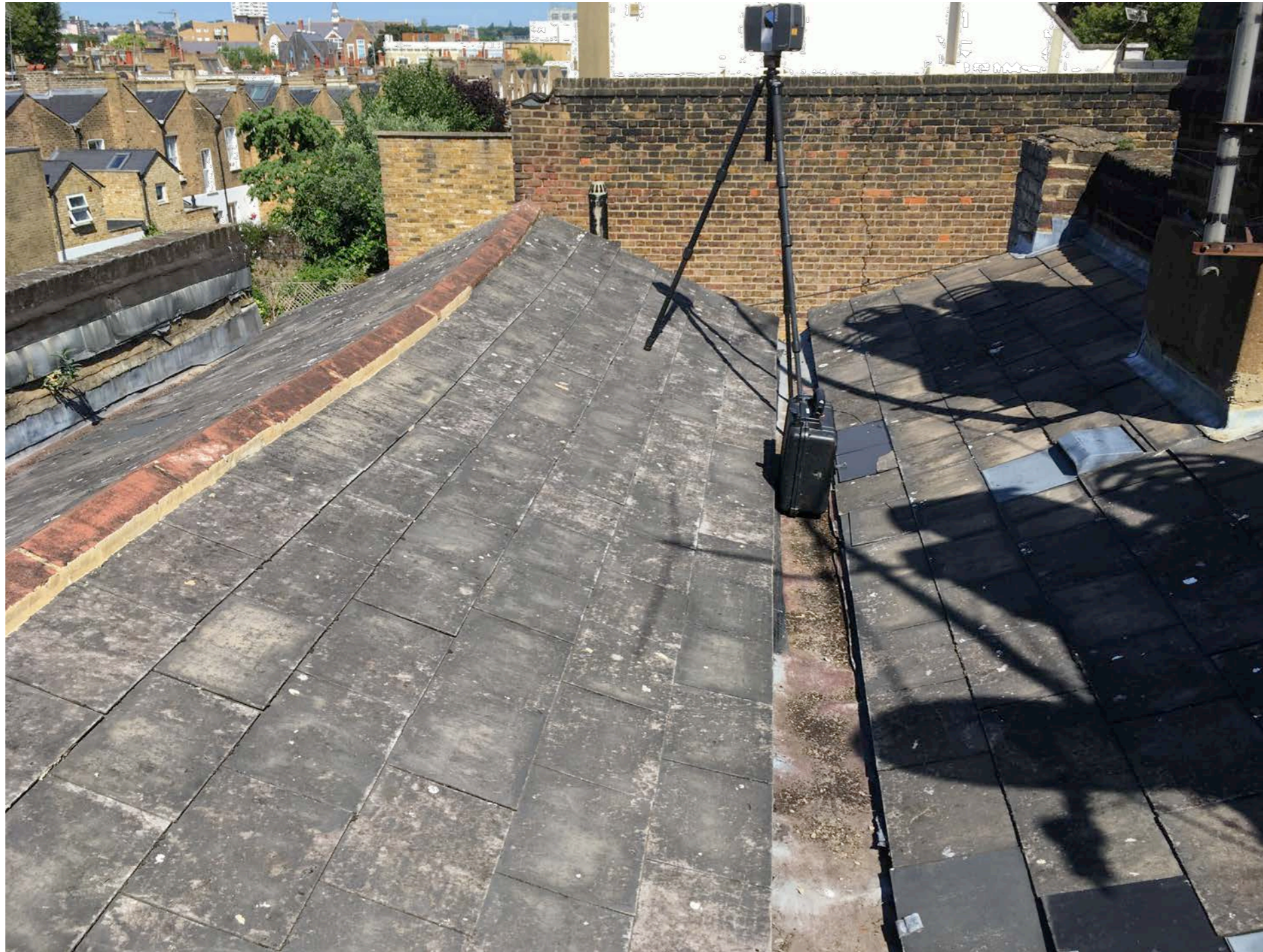
01 | Roof - View 1 (towards rear) scale N/A
