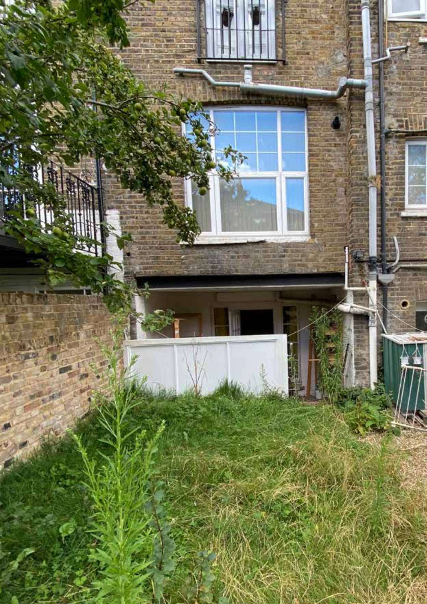
The existing elevation viewed from the rear garden
