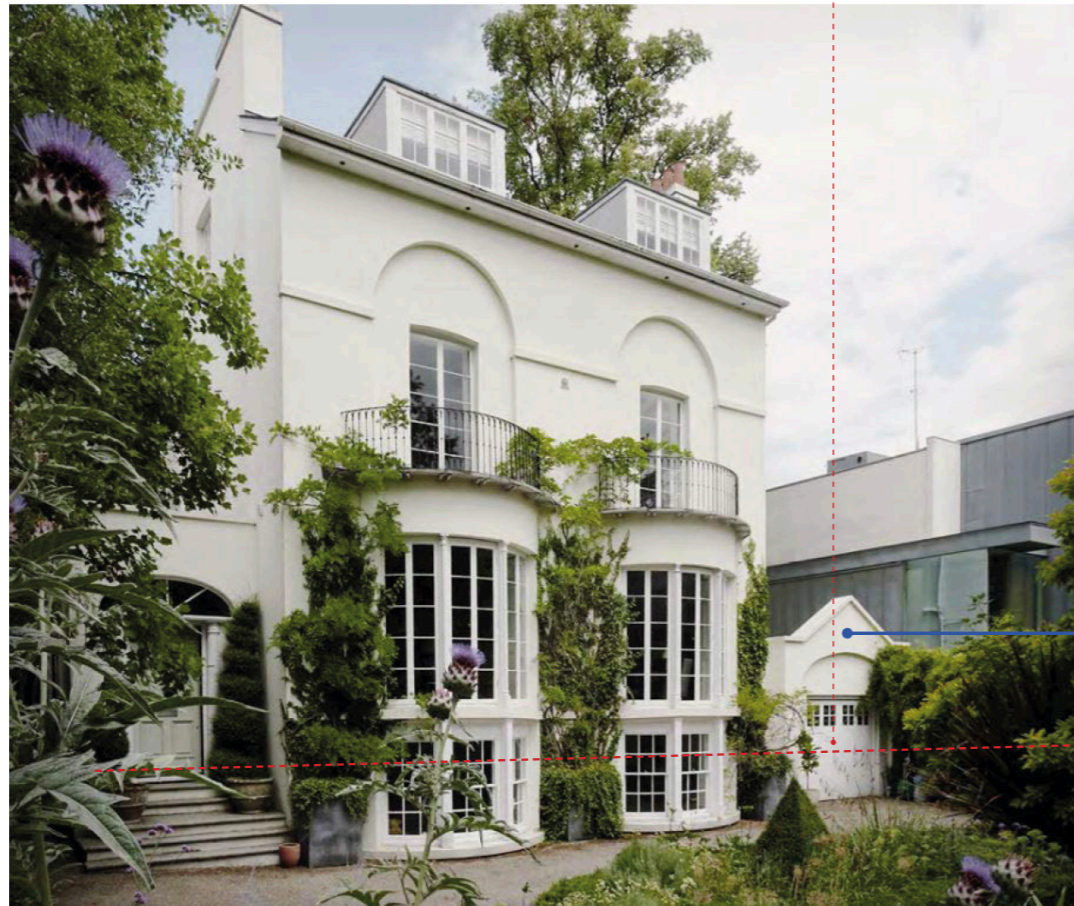
Photo of front elevation of No.12 Keats Grove.
