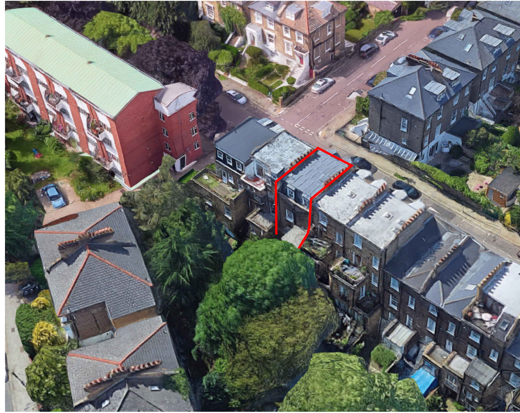
EXISTING AERIAL VIEW FROM EAST
