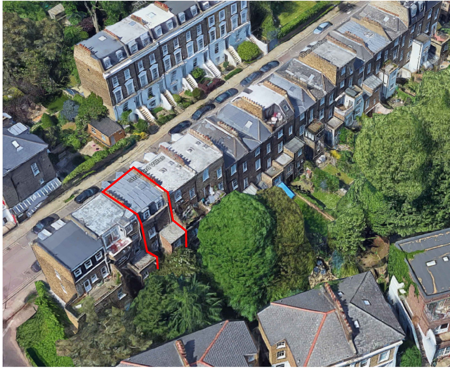
EXISTING AERIAL VIEW FROM SOUTH
