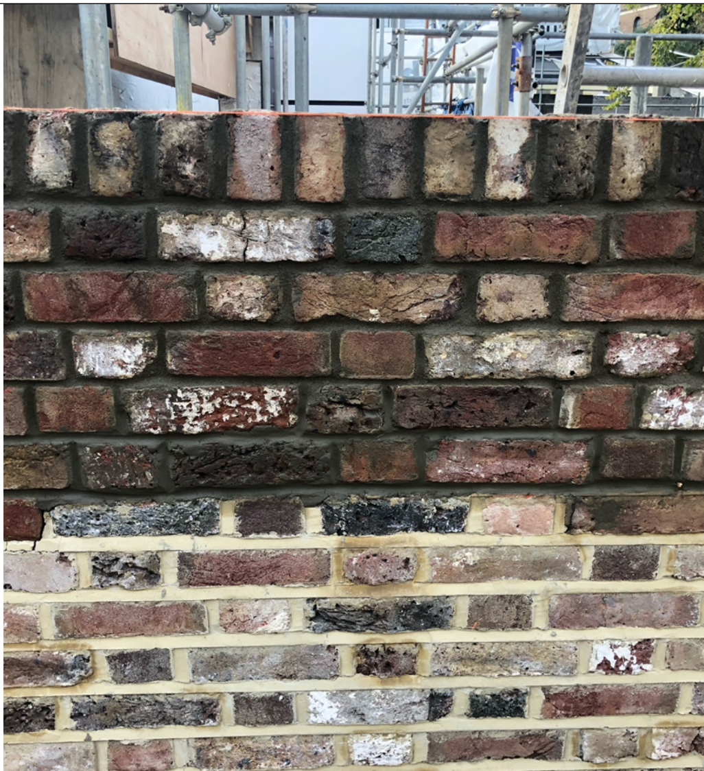
Figure 01: Sample panel showing initially submitted pointing detail to the bottom, and amended more traditional pointing to the top.
