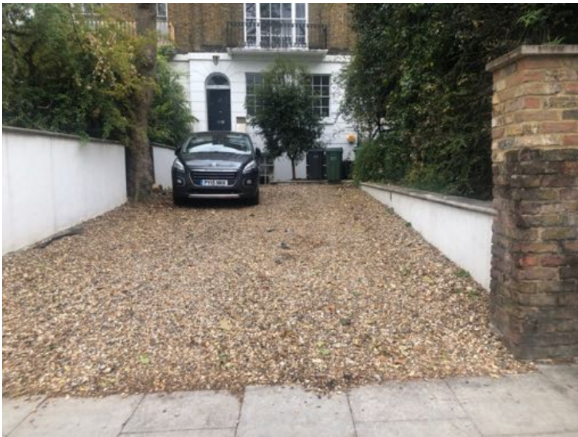
2: Existing front elevation and driveway
