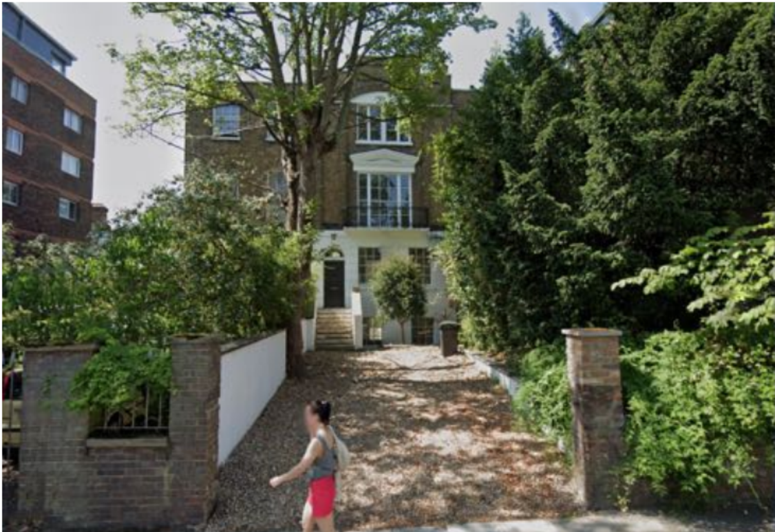
1: Existing front elevation and driveway
