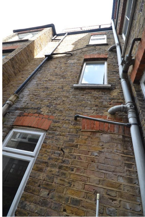
Side existing window previously blocked, to be opened).
