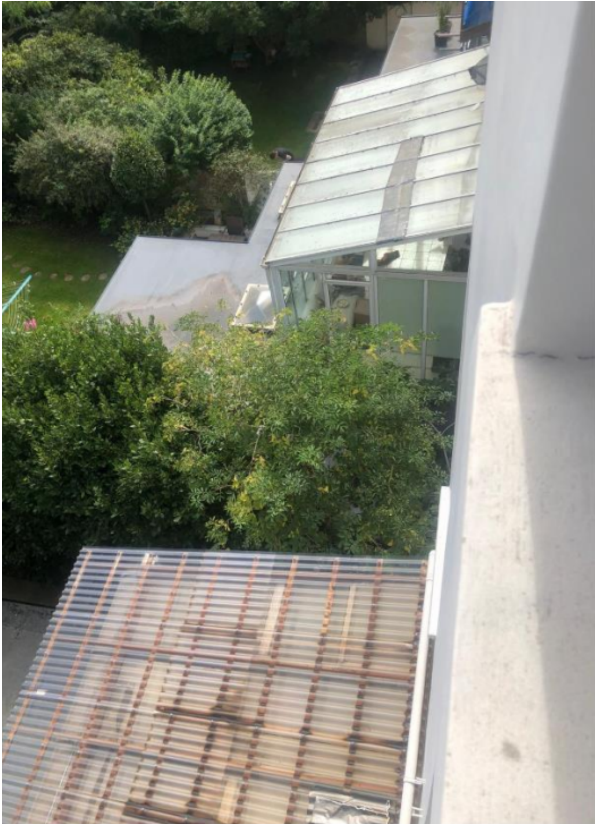
Figure 3: The existing roof of the structure alongside the neighbouring property
