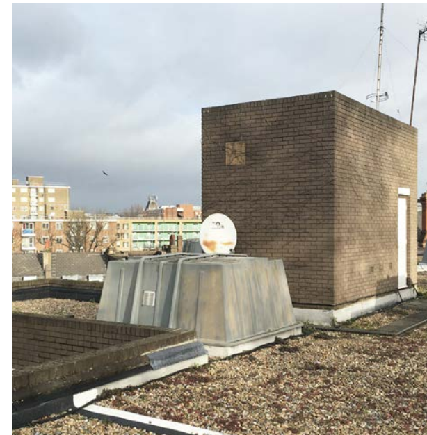
Roof level lift shaft
