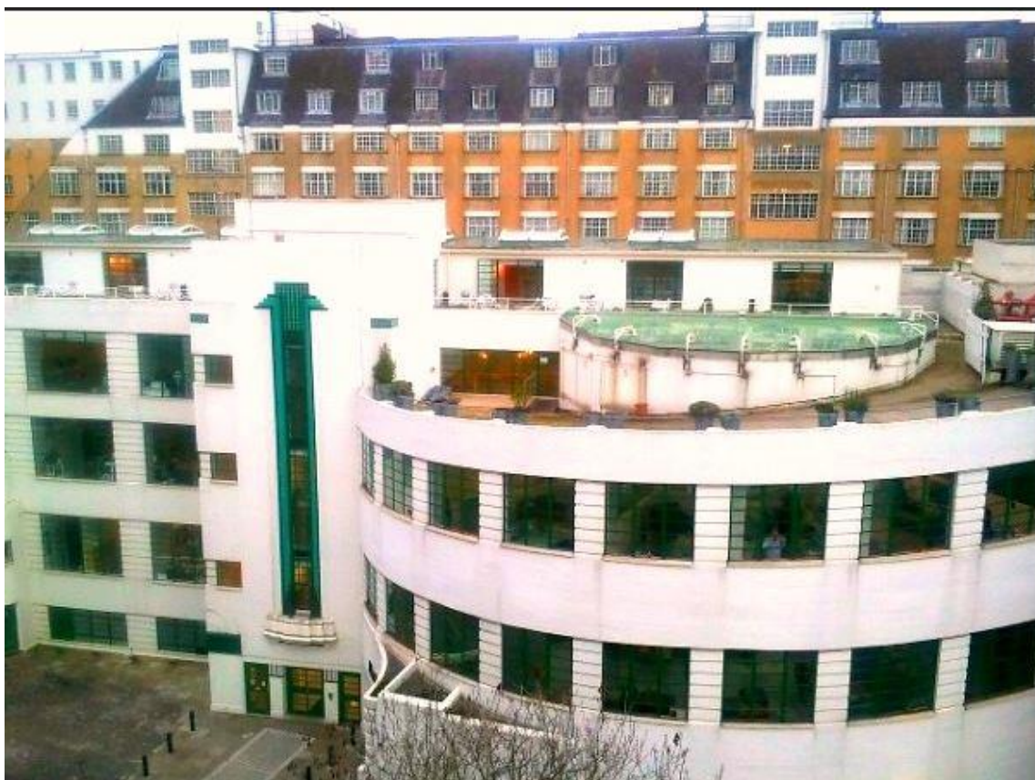
Figure 5 Former Daimler Garage, main frontage, c. 1990s
