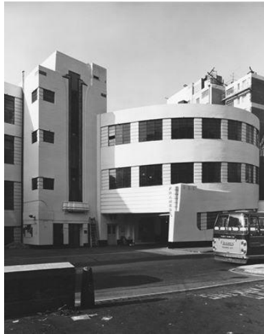
Figure 12 Former Daimler Garage main frontage, c.1970s
