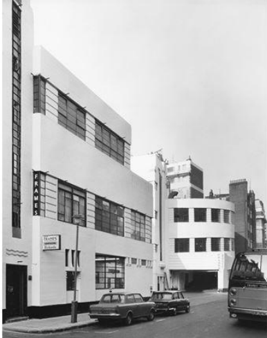
Figure 9 Former Daimler Garage main frontage, c.1970s
