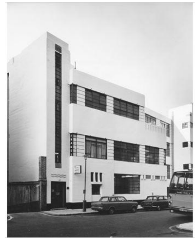
Figure 13 Former Daimler Garage main frontage, c.1970s
