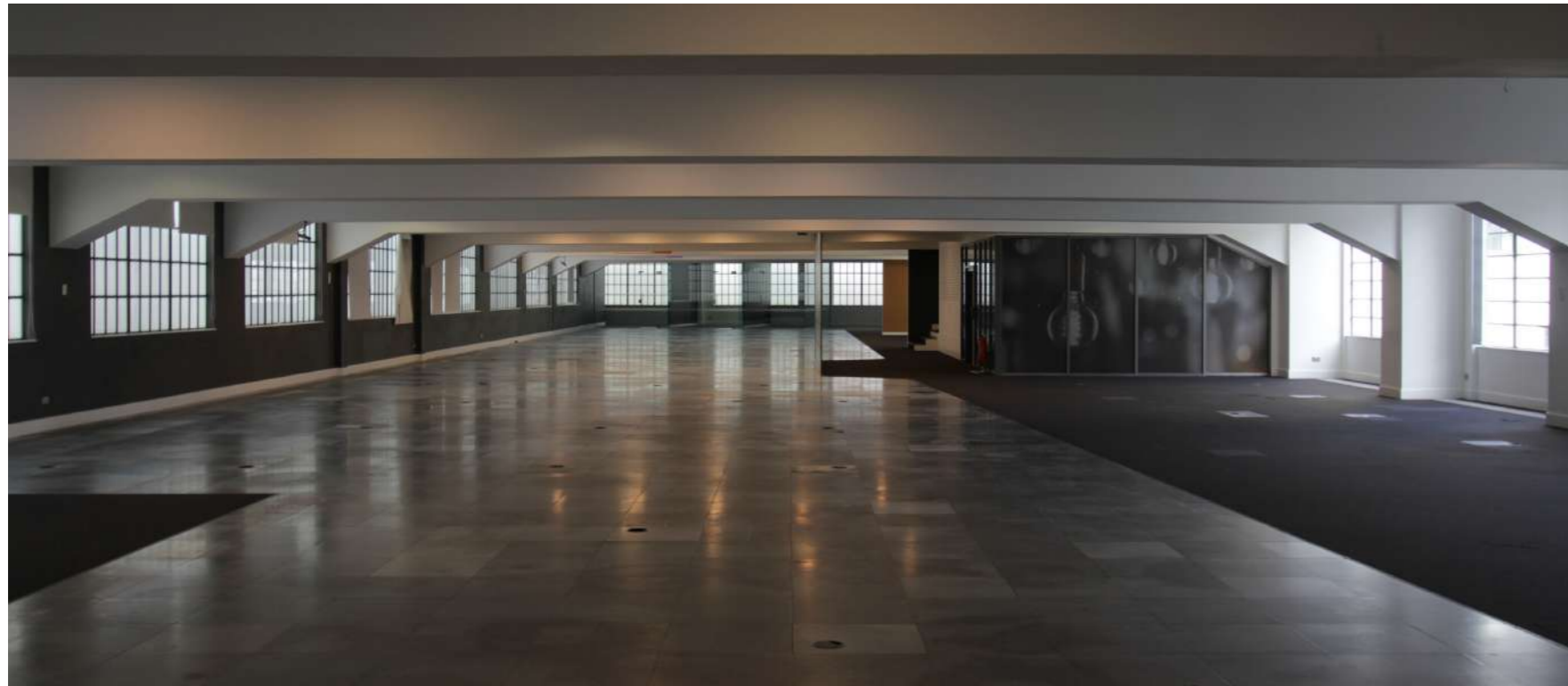
Existing window treatment on a typical floor
