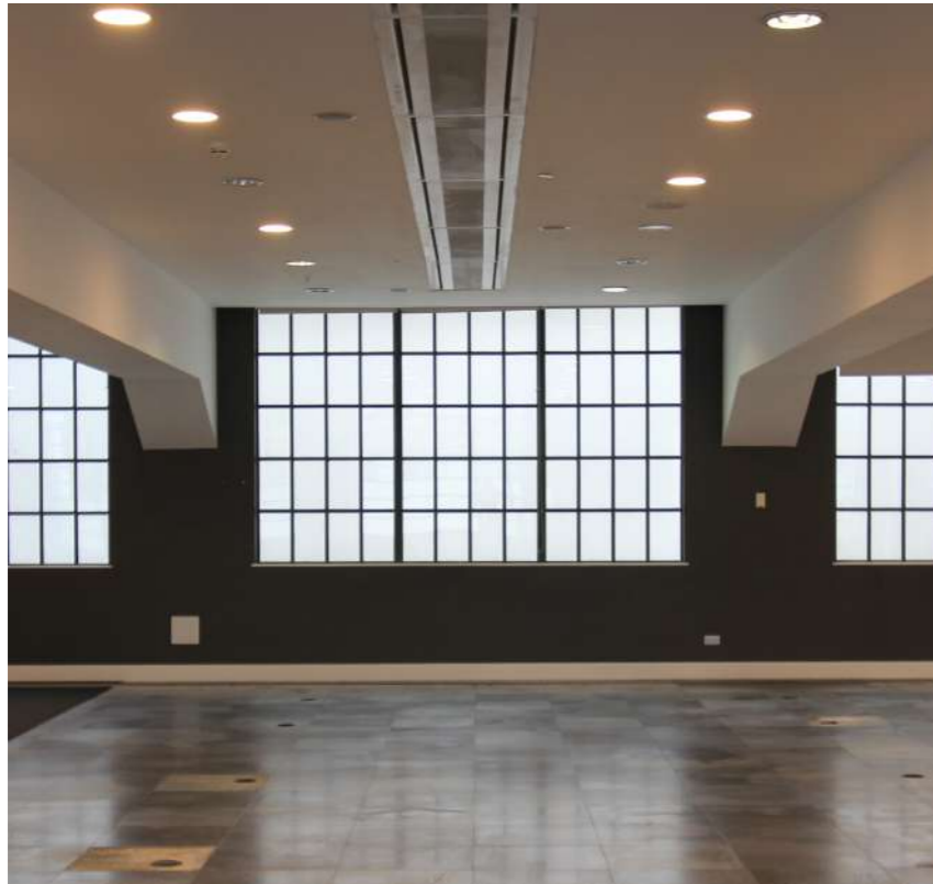
Existing window treatment - level 02
