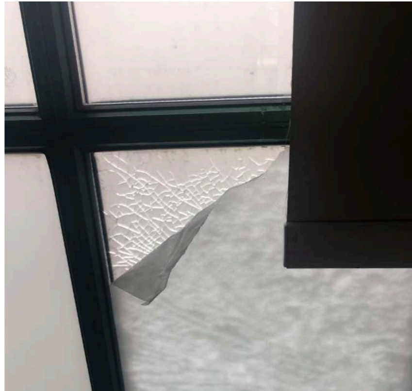
Existing film on windows
