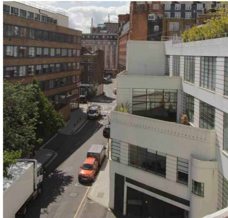
02. View from the top of the ramp looking south
