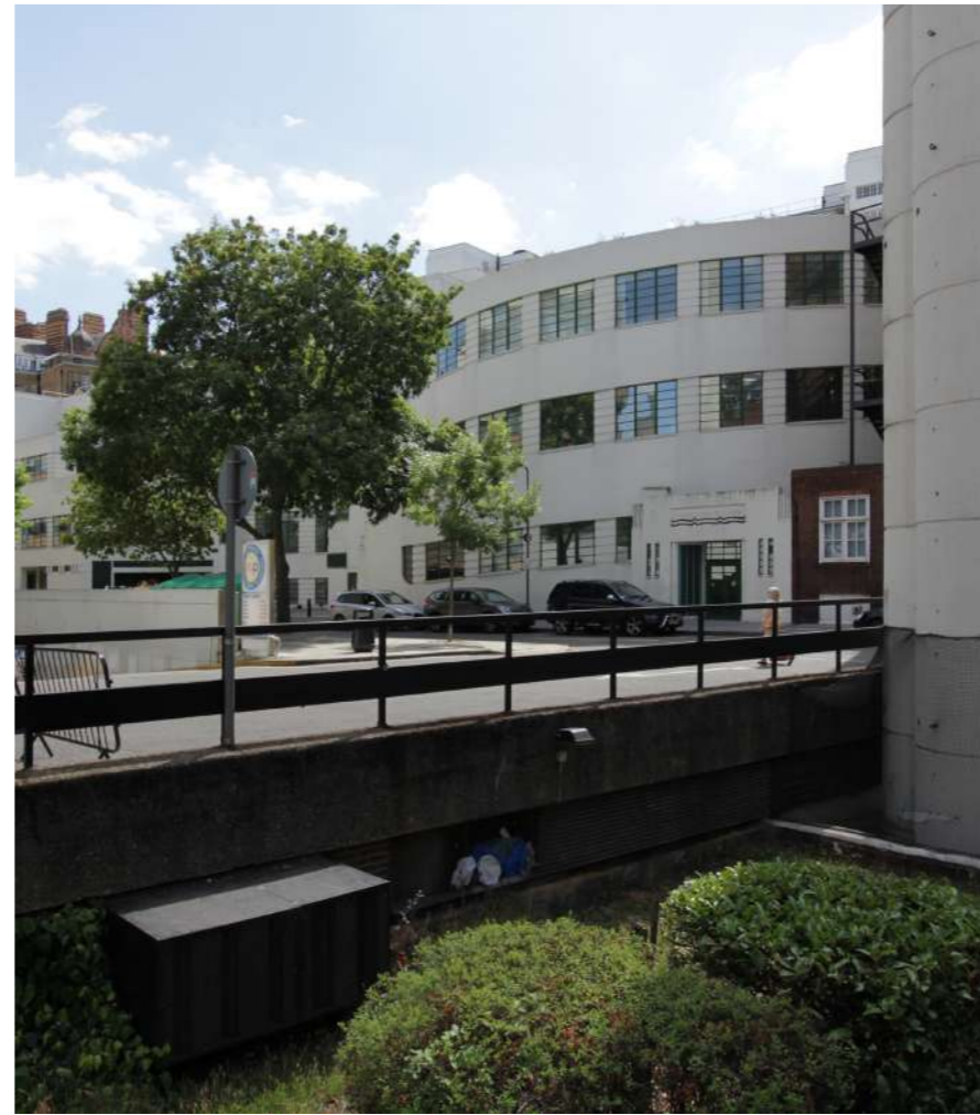
View from Coram Street (looking south)
