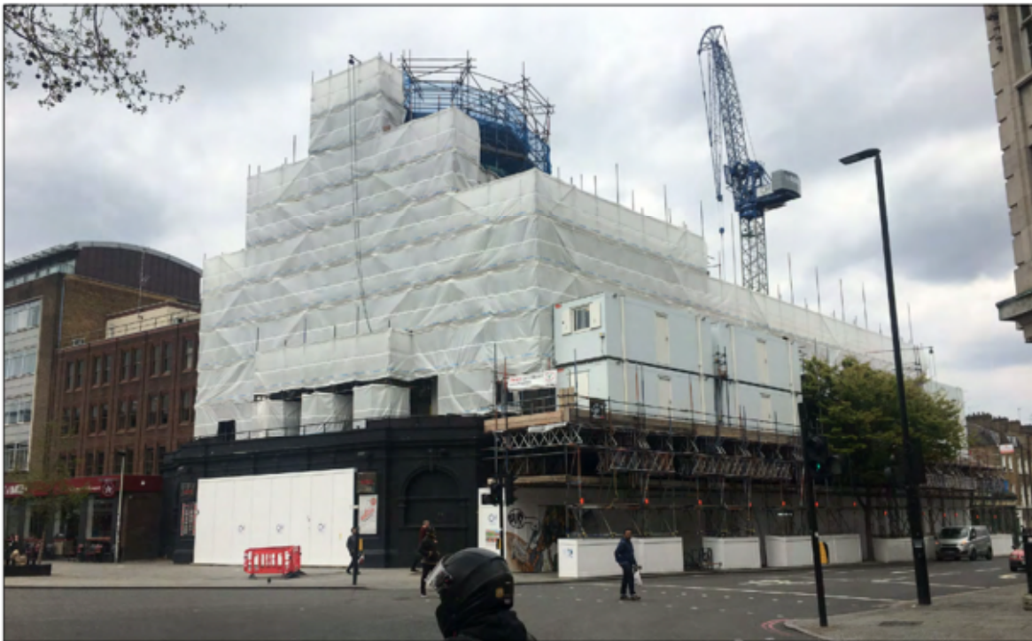
1. Existing view of scaffolding
