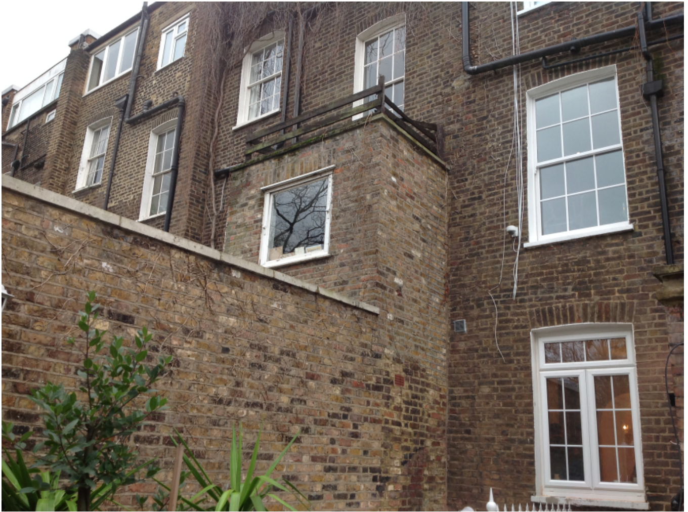
Side flank of no. 32's extension
