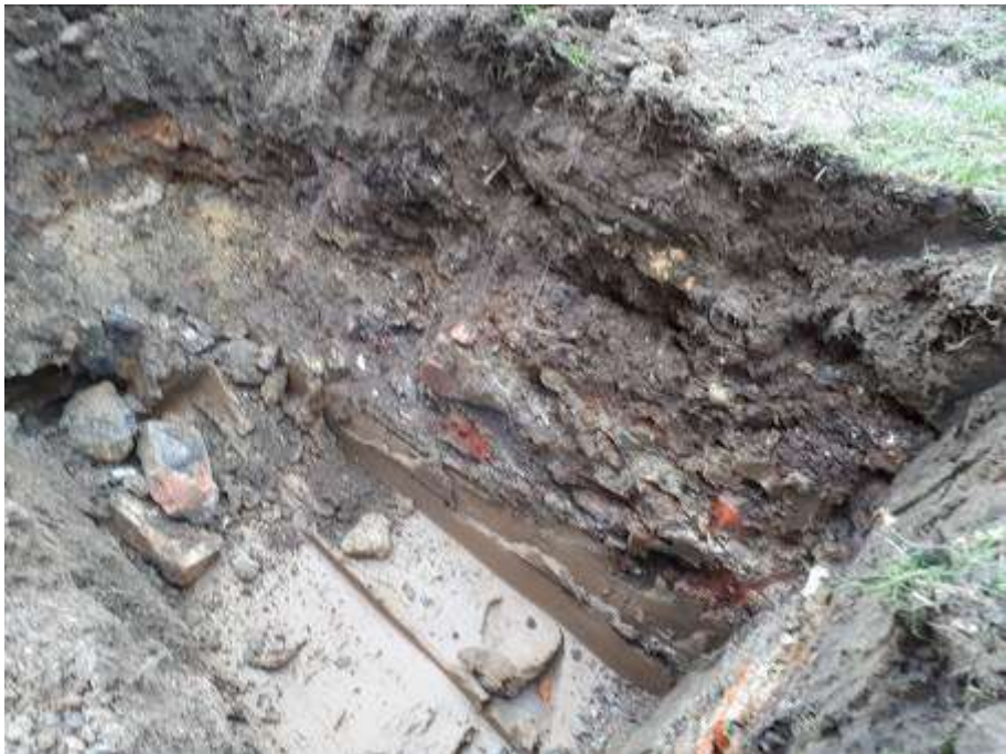
Plate 8 Showing excavation at HP06
