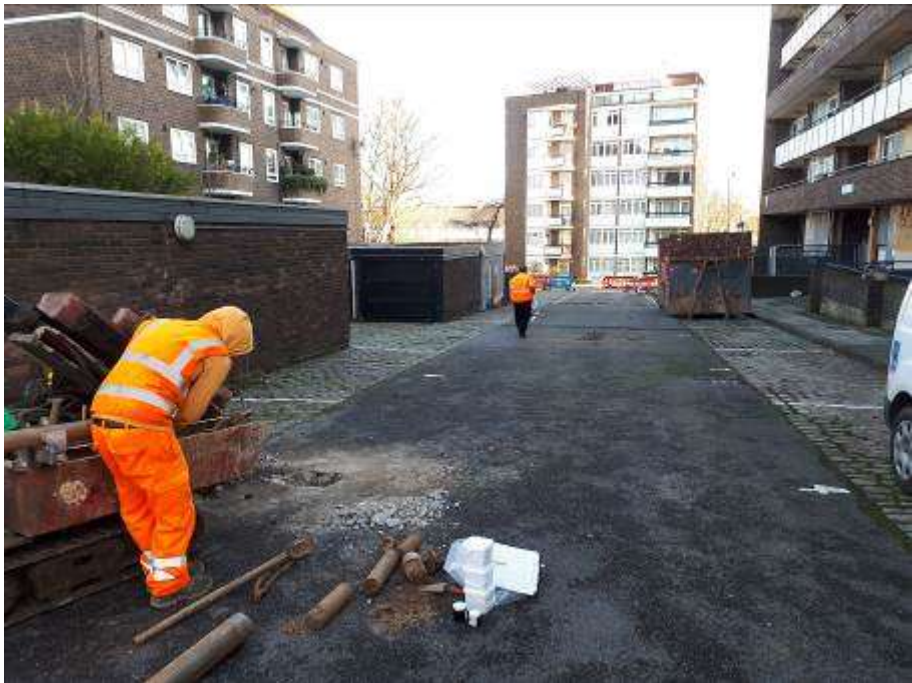
Plate 2 Showing location of window sample WS02 within Aspen House
