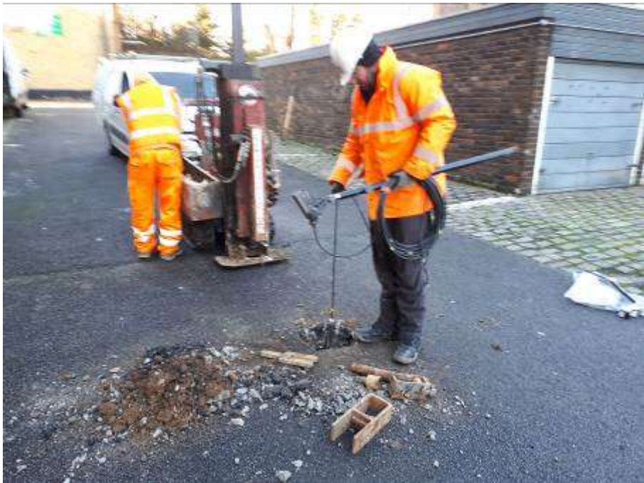
Plate 1 Showing EOD engineer assessing risk within window sample hole
