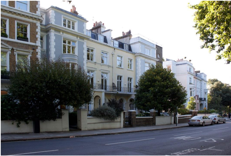
106-108 Front Elevation: Existing Colour
