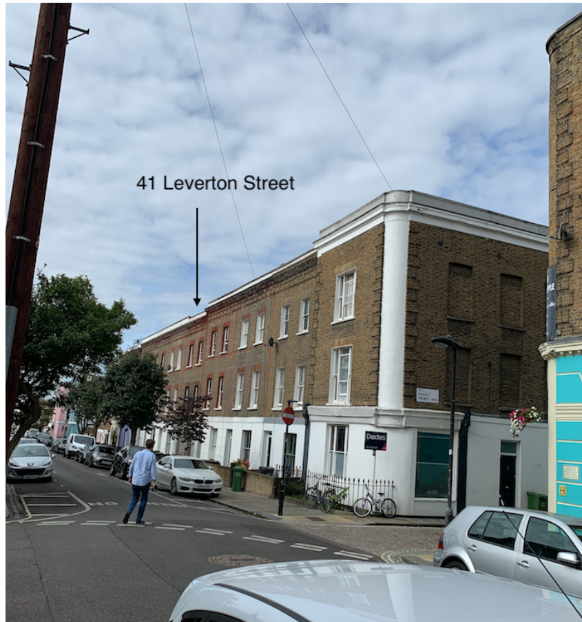
View of 41 Leverton Street from the north at junction with Railey Mews
