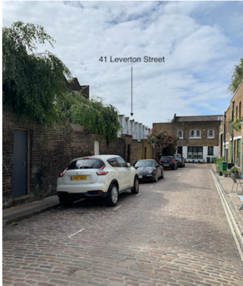
View of rear elevation of the block containing 41 Leverton Street taken from outside 5 Railey Mews
