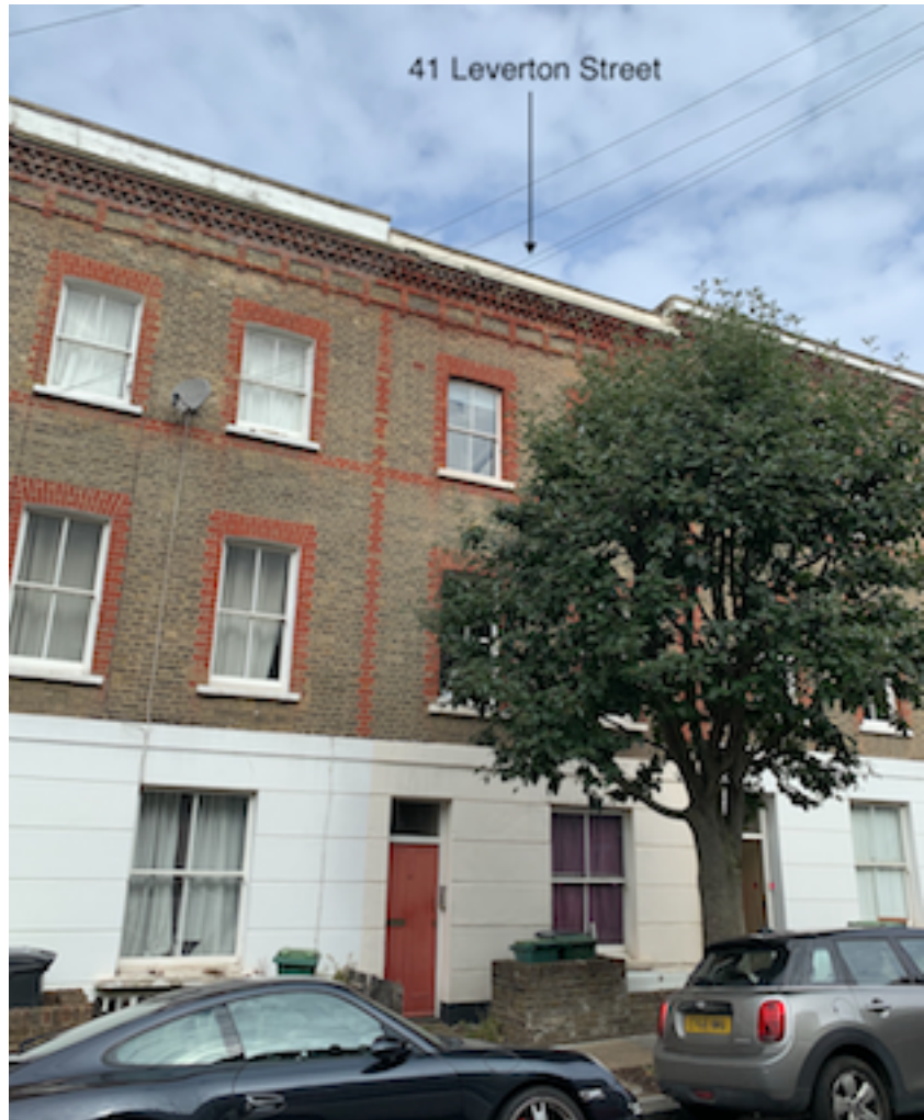
View of 41 Leverton Street
