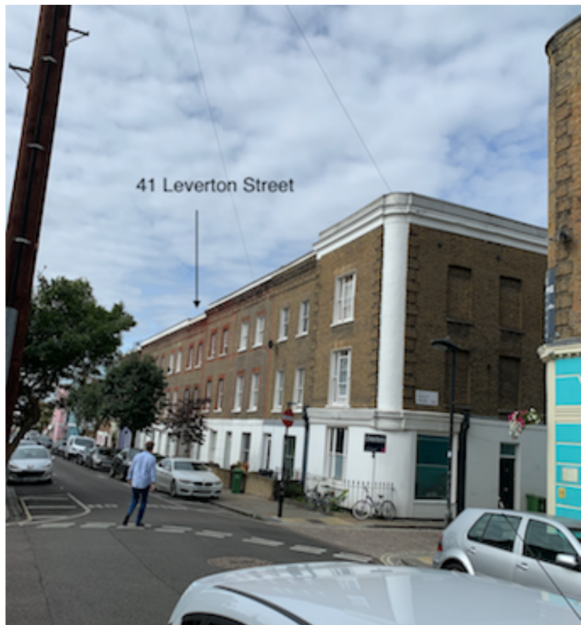
View of 41 Leverton Street from north at junction with Railey Mews
