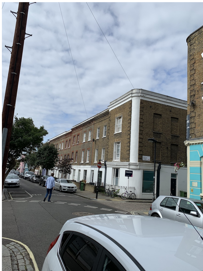
Existing View along Leverton Street
