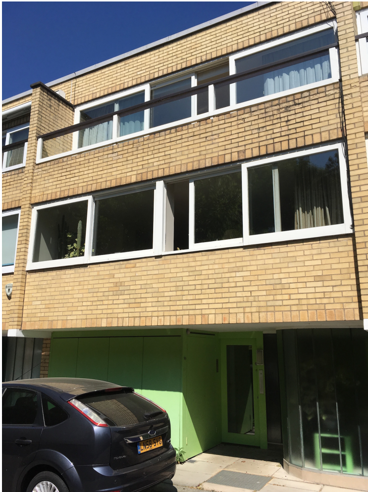
Photo 1: The front elevation showing the entrance at the Lower Ground Level
