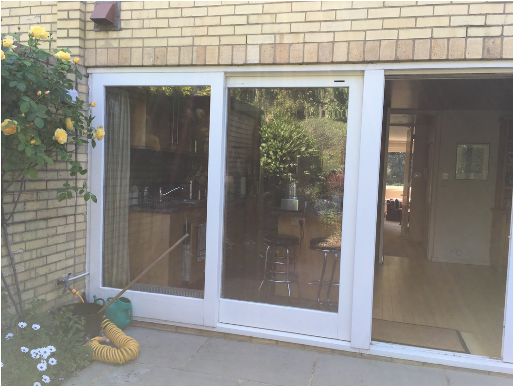
Photo 4: Kitchen windows viewed from Rear Garden
