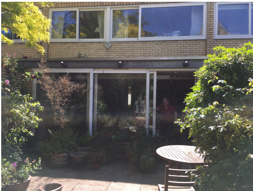
Photo 6: View of 95 Swains Lane, seen from rear garden.
