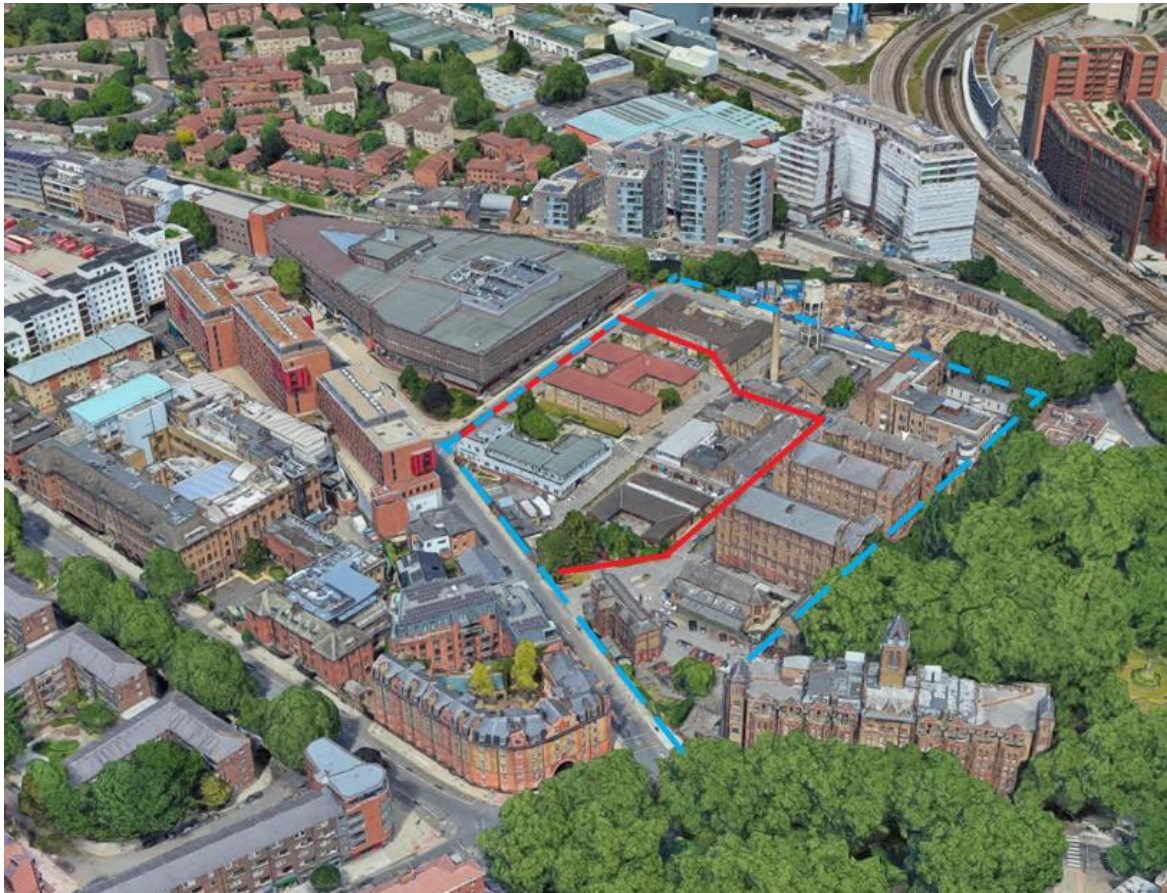
Figure 2-1 Red line showing the extent of the plot where Proposed Building will be located within the wider St Pancras Hospital Site
