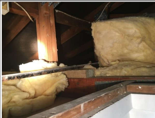
Photo 5. Roof void of Jules Thorn Day Centre (B1).
