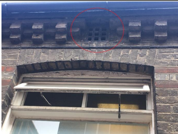
Photo 16. Shallow grill on the Kitchen Block (B6).
