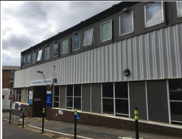
Photo 11. Southern elevation of the Bloomsbury Day Centre (B4).
