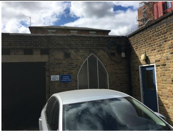
Photo 13. Flat roof on the Post Room and Former Mortuary building (B5).
