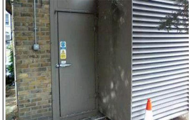
Photo 15. Generator room in the Post Room and Former Mortuary building (B5).
