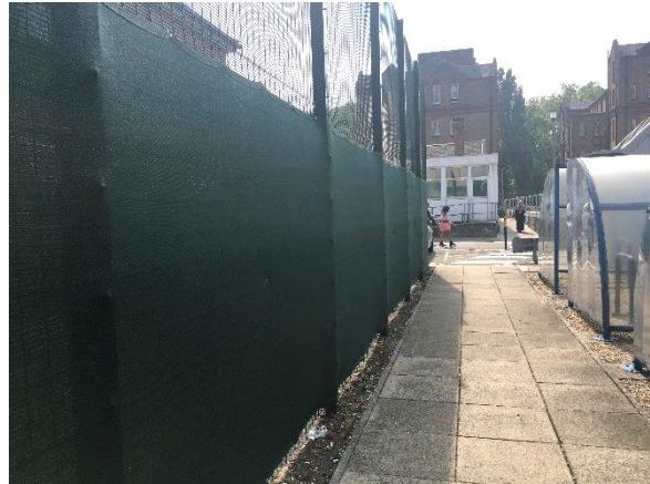
Photo D10 Security fencing around Ash House (B3)
