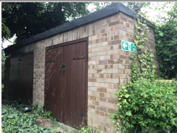
Photo 4. Brick outbuilding east of Jules Thorn Day Centre (B1) fence.
