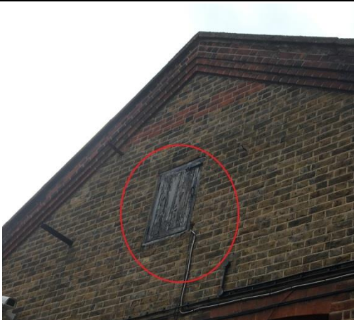
Photo 7. Airing door leading to roof void at the Camley Centre (B2).
