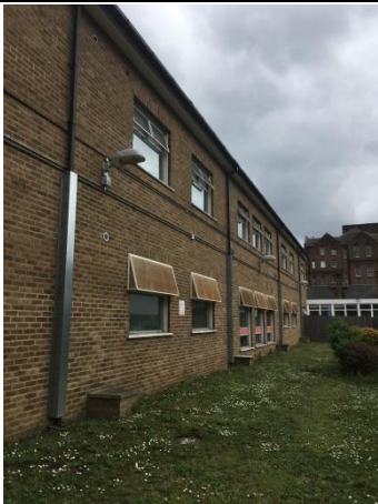
Photo 10. Eastern elevation of Ash House (B3).
